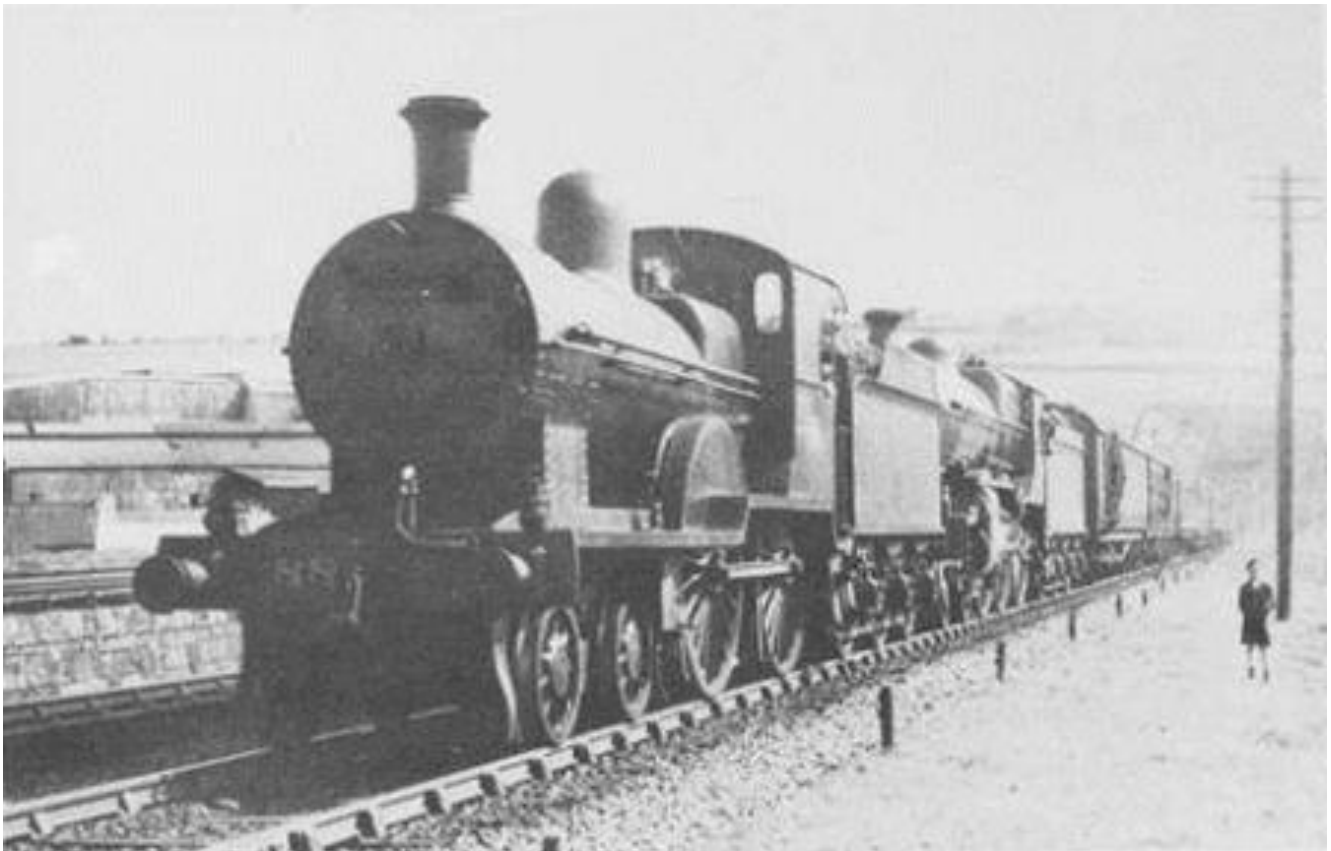
D14 No.88 with new frames, etc., and Z boiler piloting No.407 on Up Mail at Kilbarry in April 1954. (W.H.C. Kelland)
