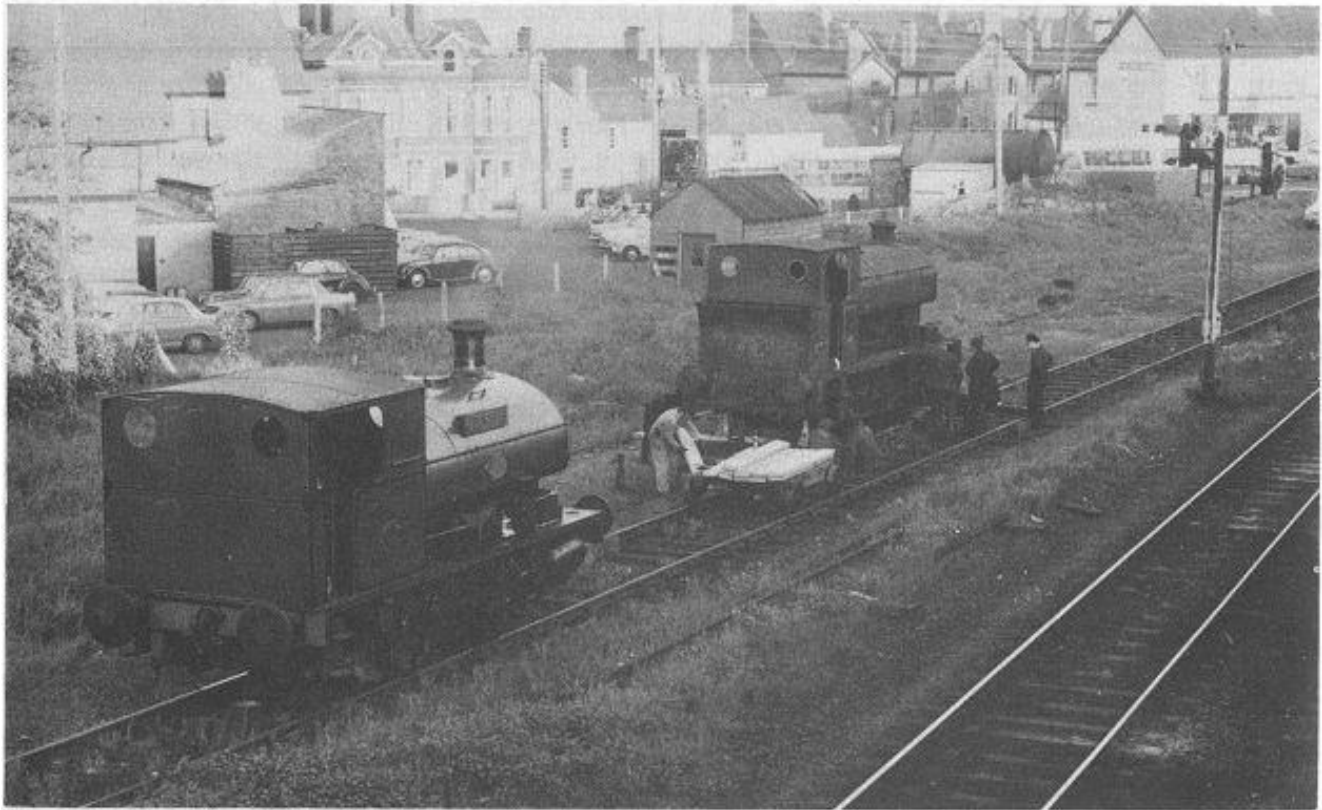
Transverse jacking of “R.H. Smyth” onto the rails at Whitehead with the “Guinness” in attendance on 10 th June 1972. (W.S. Boomer)
