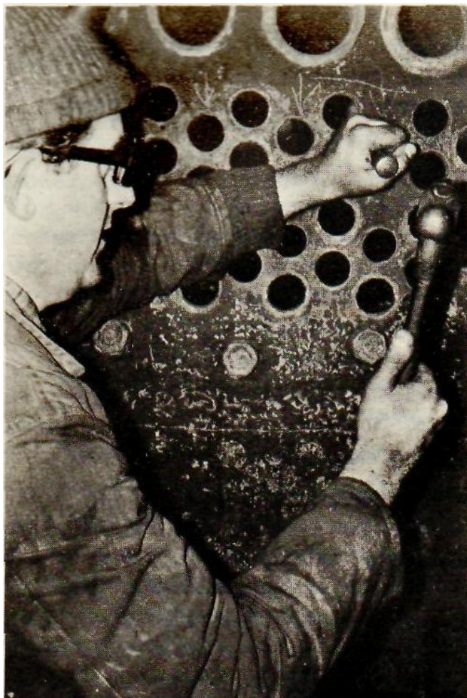
Inside No.186's firebox, Bob Edwards works at crimping the ends of the old tubes. This work is done under supervision. (C.P. Friel)
