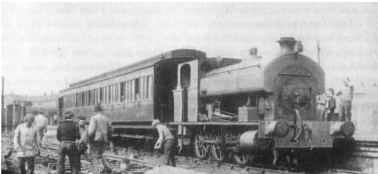
“R.H. Smyth” on Sunday train rides duty, while a track gang works at installing the new crossover. (C.P. Friel)
