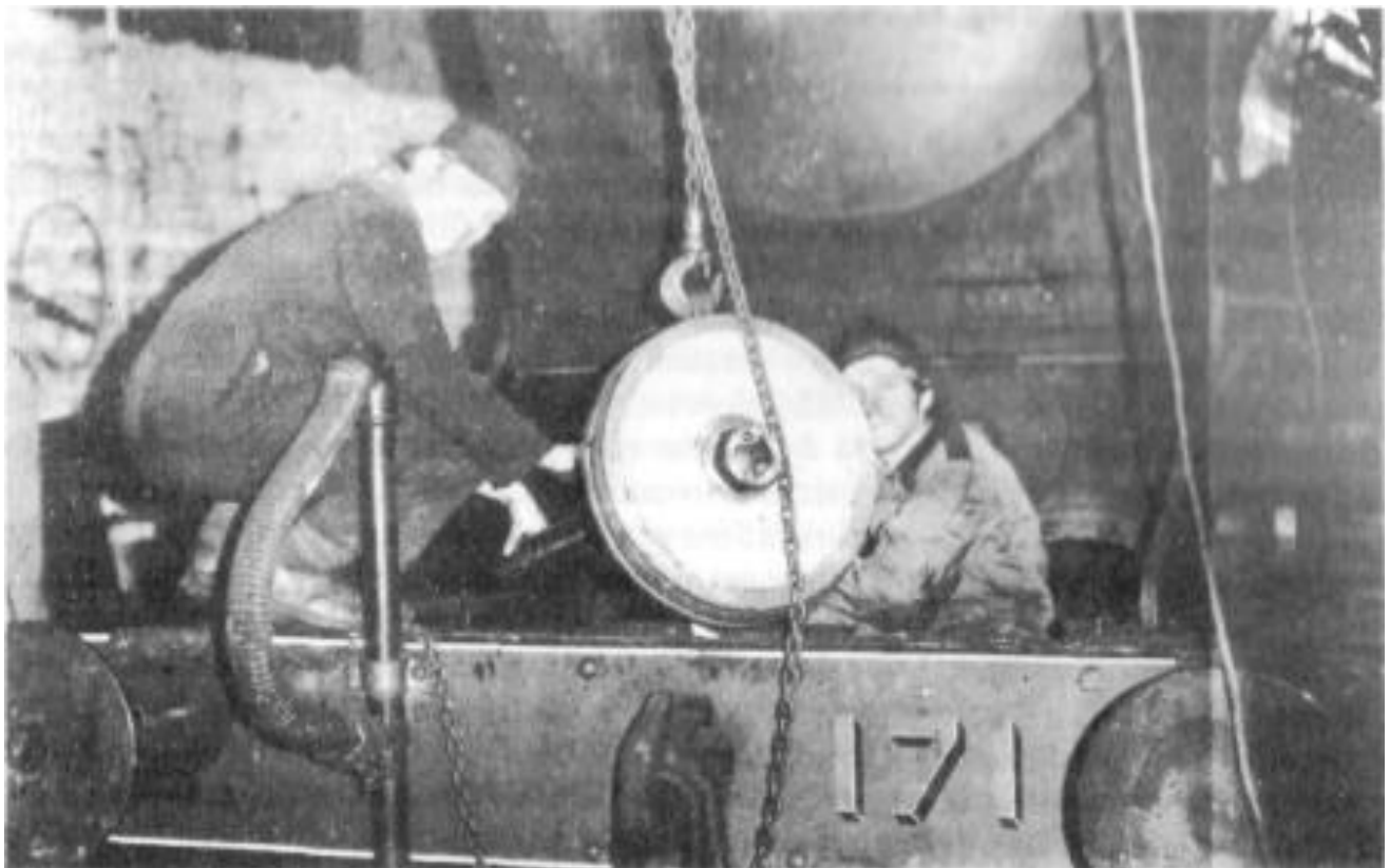
Brian Hill (left) and Paul Newell refit No.171's right-hand piston, following replacement of the piston head. (C.P. Friel)
