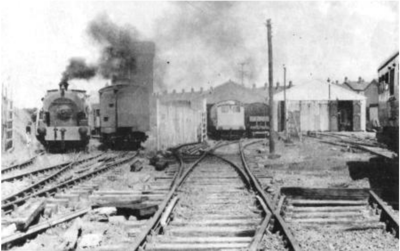
“R.H. Smyth” is in No.1 carriage siding. In the centre can be seen the turnout which will eventually lead to the heavy lifting area, while the track on the right will be joined to the point work in front of the new shed to form the eight coach run round. (C.P. Friel)
