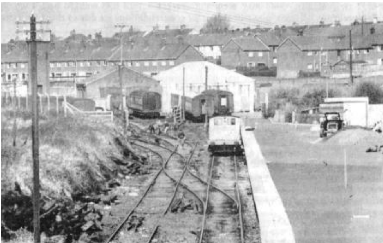
A telephoto shot from the King's Road bridge shows the new point work immediately after the crossover was installed last year. The tracks to the left lead to the carriage yard. (C.P. Friel)
