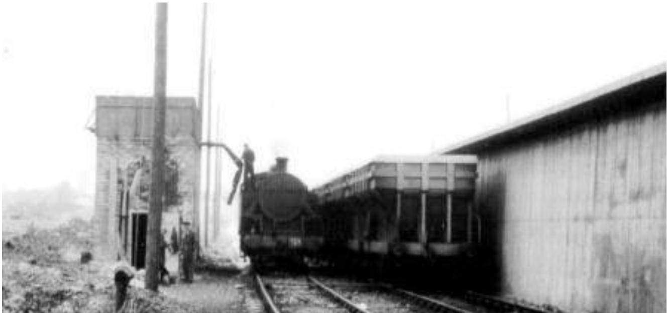
No.51 at the water tank at Magheramorne. One of the two loading banks is on the right, while the “lop-sided” construction of the stone wagons shows clearly. (W.T. Scott)
