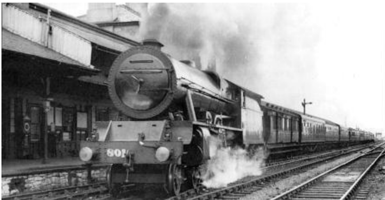
No.801 “Macha”, with burned smokebox door, on the 10:30am from Kingsbridge to Cork and Kerry. This train will divide at Mallow, the Killarney and Tralee portion probably being worked forward by a 321 class 4-4-0. Few CIÉ engines carried a lamp iron on the smokebox but that on 801 was for the headboard of the short-lived Belfast - Dublin - Cork Enterprise. (Kelland Collection)
