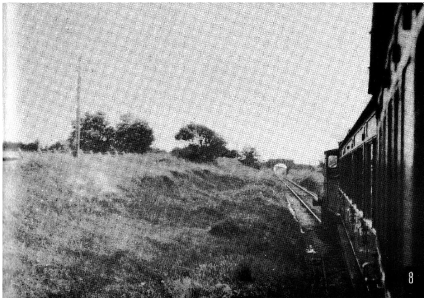
TUBBERCERRY: Behind D14 class 4-4-0 No.95 (Inchicore 1885) on the 4:40pm Sligo to Limerick on 29 th June 1938. This is a fairly typical bit of Burma Road with minimum earthworks and the line following the contours of the ground in short, sharp banks. (H.C. Casserley)
