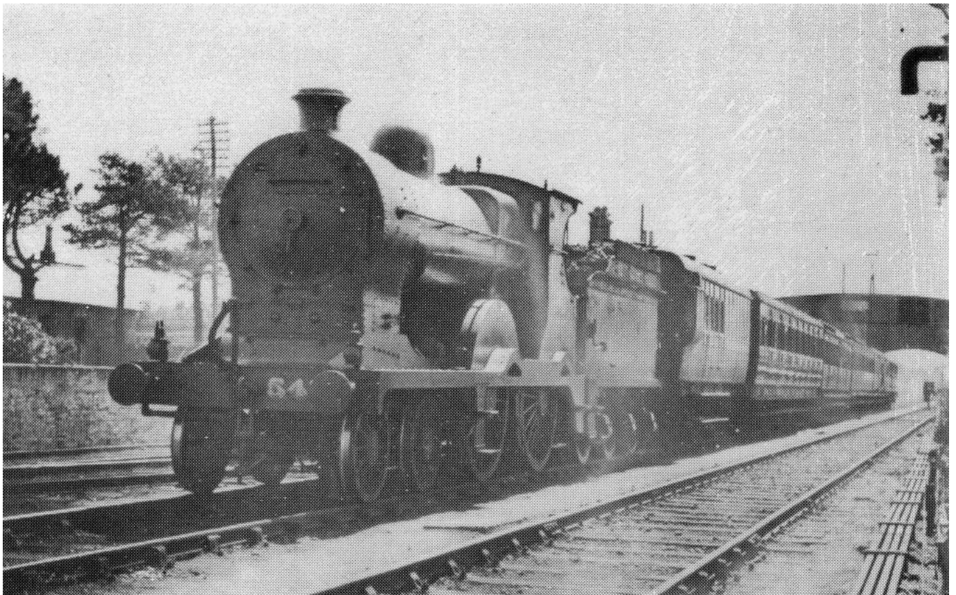
D6 class 4-4-0 No.542 pauses at Dromod with a Sligo-bound passenger train in 1949. Note the tablet snatcher on the side of the tender. Another Broadstone product, this engine was No.9 "Kylemore" before 1925. Part of the Cavan & Leitrim's terminus can be seen on the left. (Locomotive & General, 19118)
