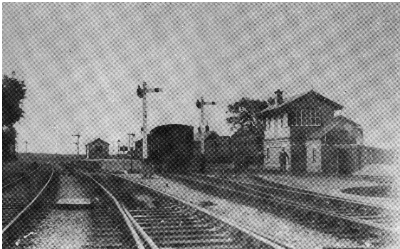
Kilfree Junction looking towards Boyle about 1933. The main line is on the left and the branch, with its turntable, is on the right. (Real Photographs, X6711)
