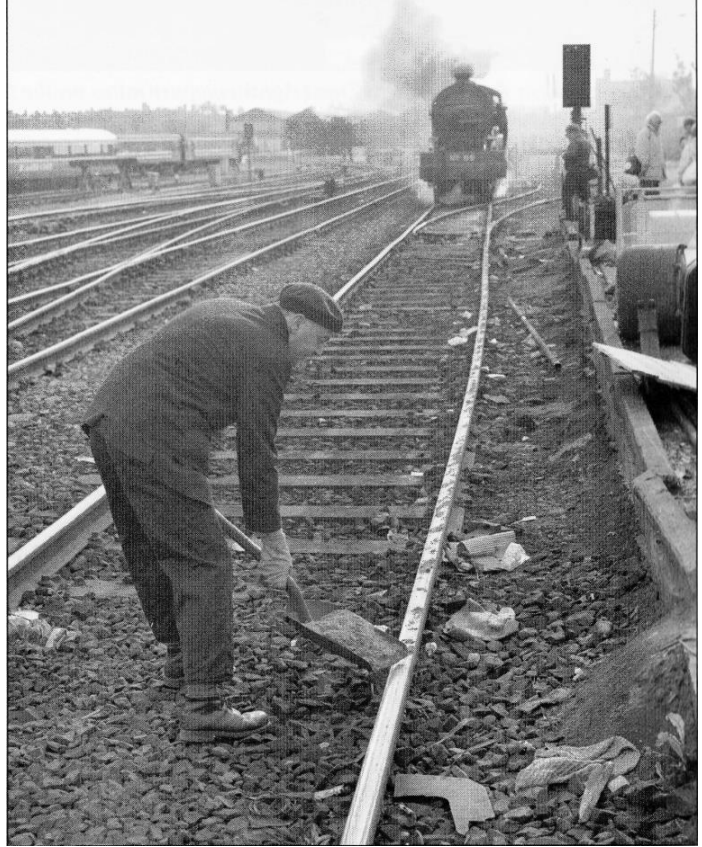
Philadelphia?: Dan Renehan sands the rails ahead of No.85 Merlin so that brother Tony will be better able to get the train out of the Military Platform. The train is the Mount Brandon Railtour which the Compound worked as far as Mallow on Saturday 14 th May 1989. CPF8905A
