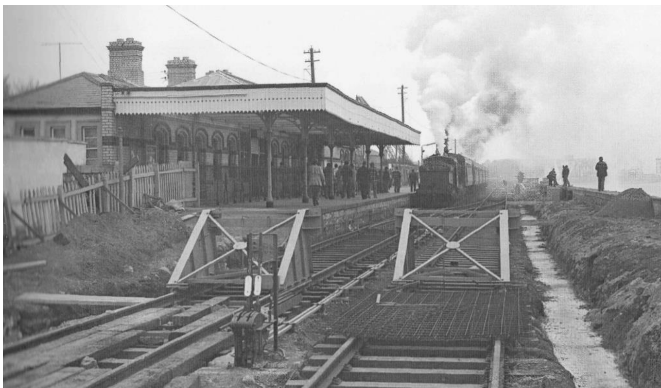
Howth: No.184 blows off as she waits to run round the train on one of her visits here on Sunday 13 th April 1980. Note the foundations for the new Down platform on the right and the two-lever ground urn to control the turnouts of the engine release. (Joe Cassells)
