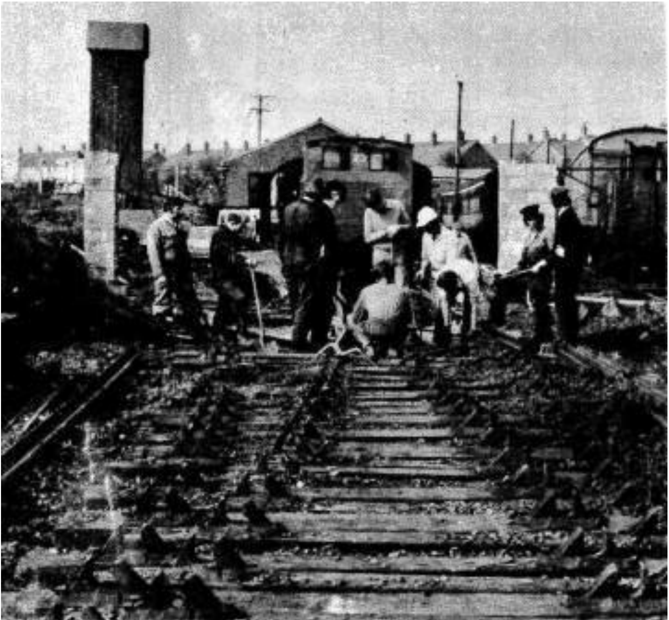
Carriage siding turnout being put in. (C.P. Friel)
