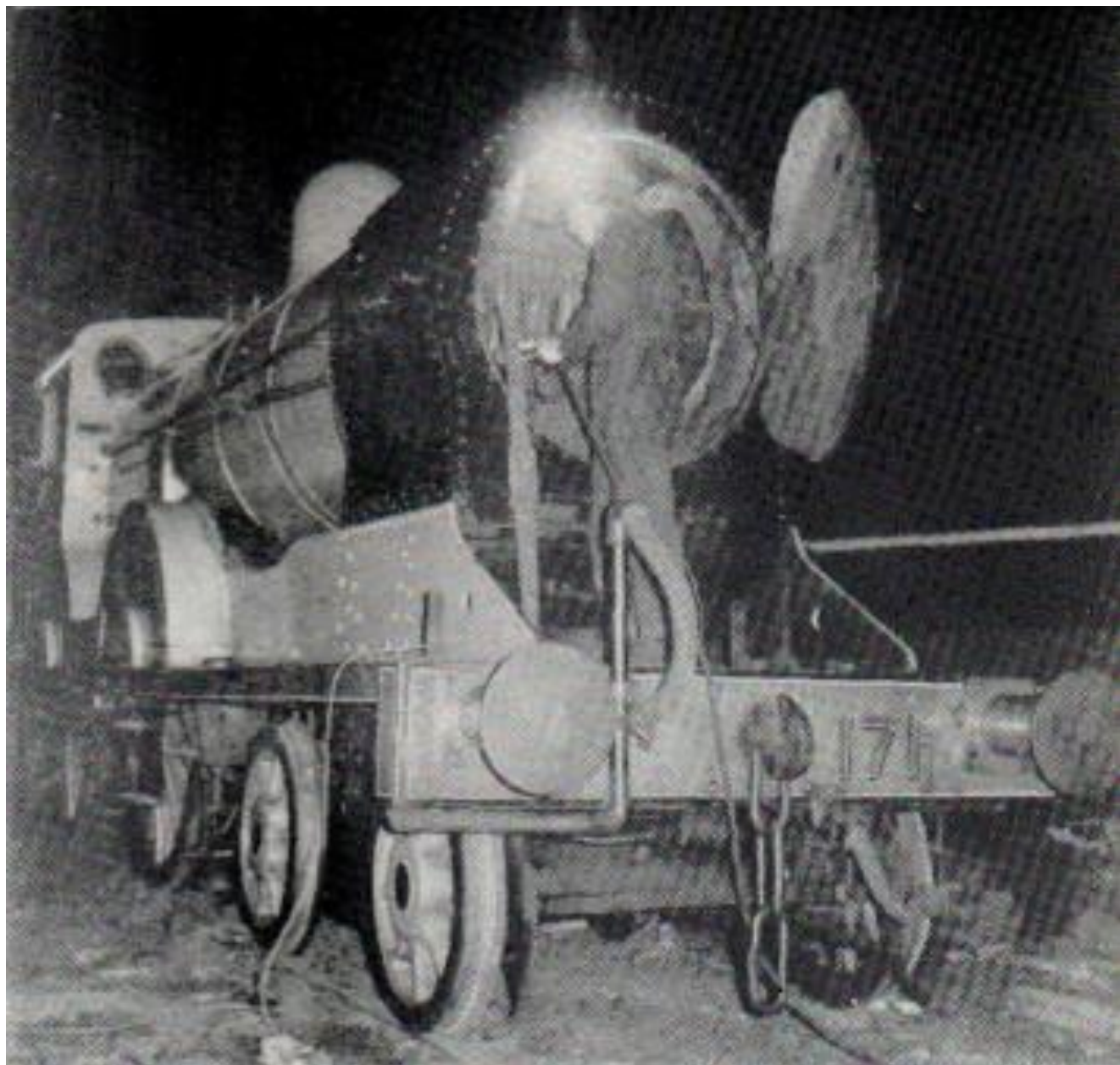
BALLYMENA & LARNE (1): No.171 started the operating season by working the “Ballymena & Larne” on 5 th April. Here we see the engine having its small tubes blown through with the compressed air line on the night before the tour. (C.P. Friel)
