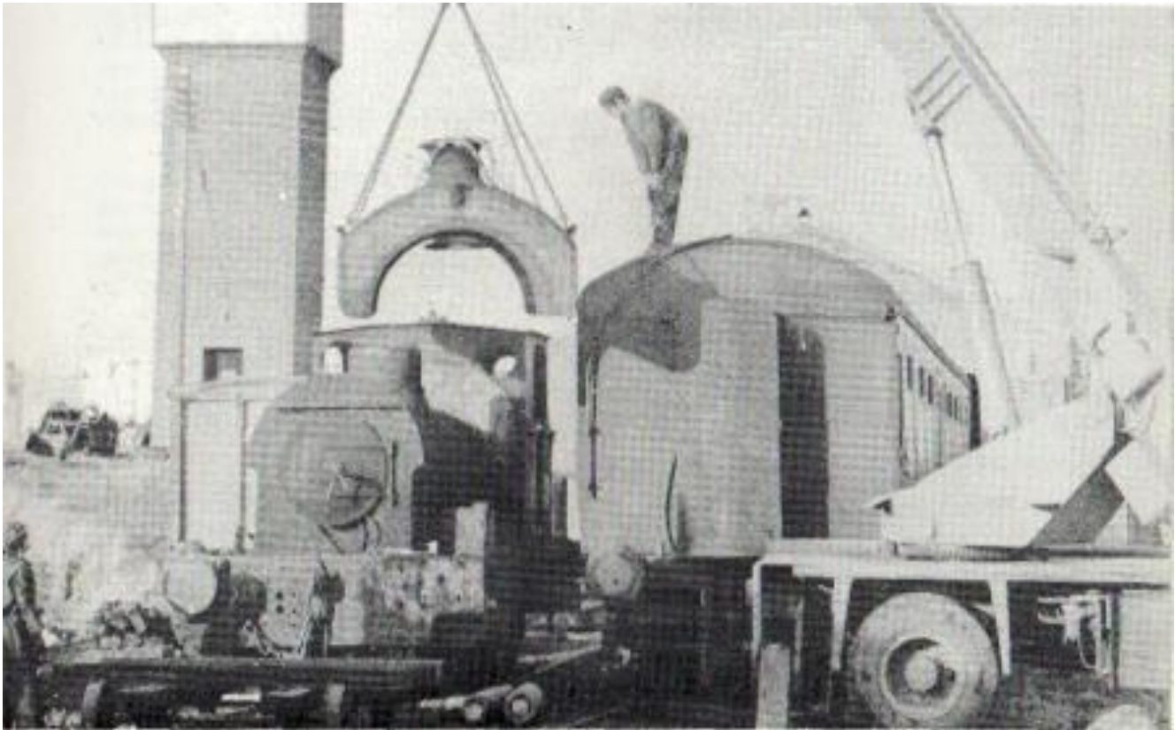
Removing the tank and chimney of "R.H. Smyth" using a hired road crane. (C.P. Friel)
