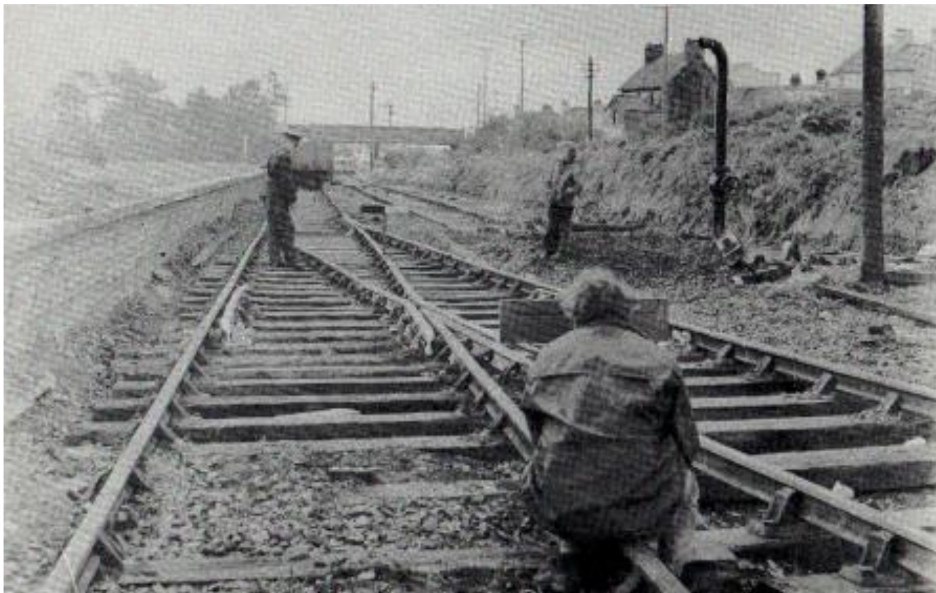
Taking levels on the newly-installed point in the platform road, giving access to the shed roads 1 and 2. The truncated 'main line' in the background has been slewed behind the water column to lead to the new No.1 Carriage Siding. (C.P. Friel)
