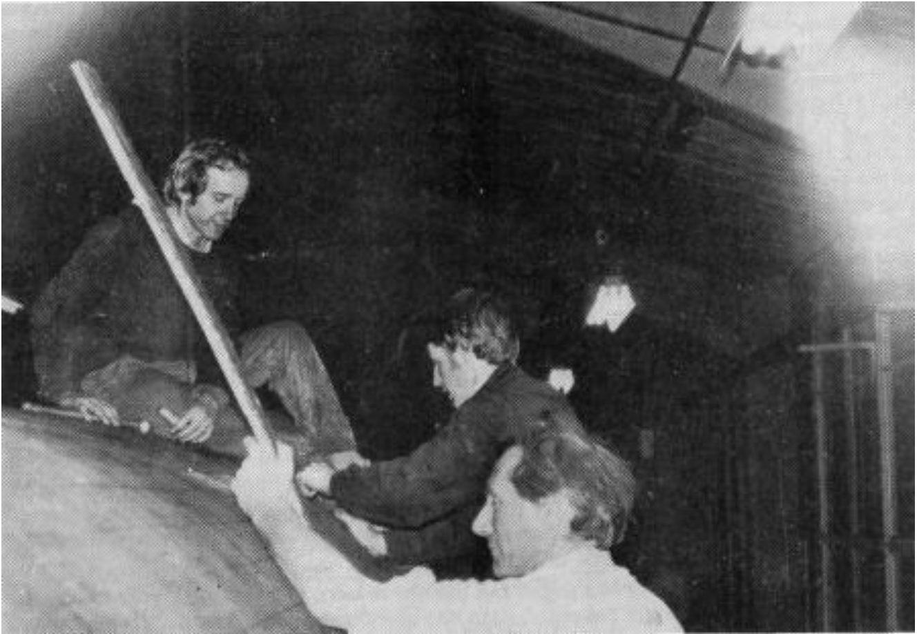
Replacing rotten timber on 550's roof. Left to right: Paul Newell, Dermot Mackie, Ken Pullin. (C.P. Friel)
