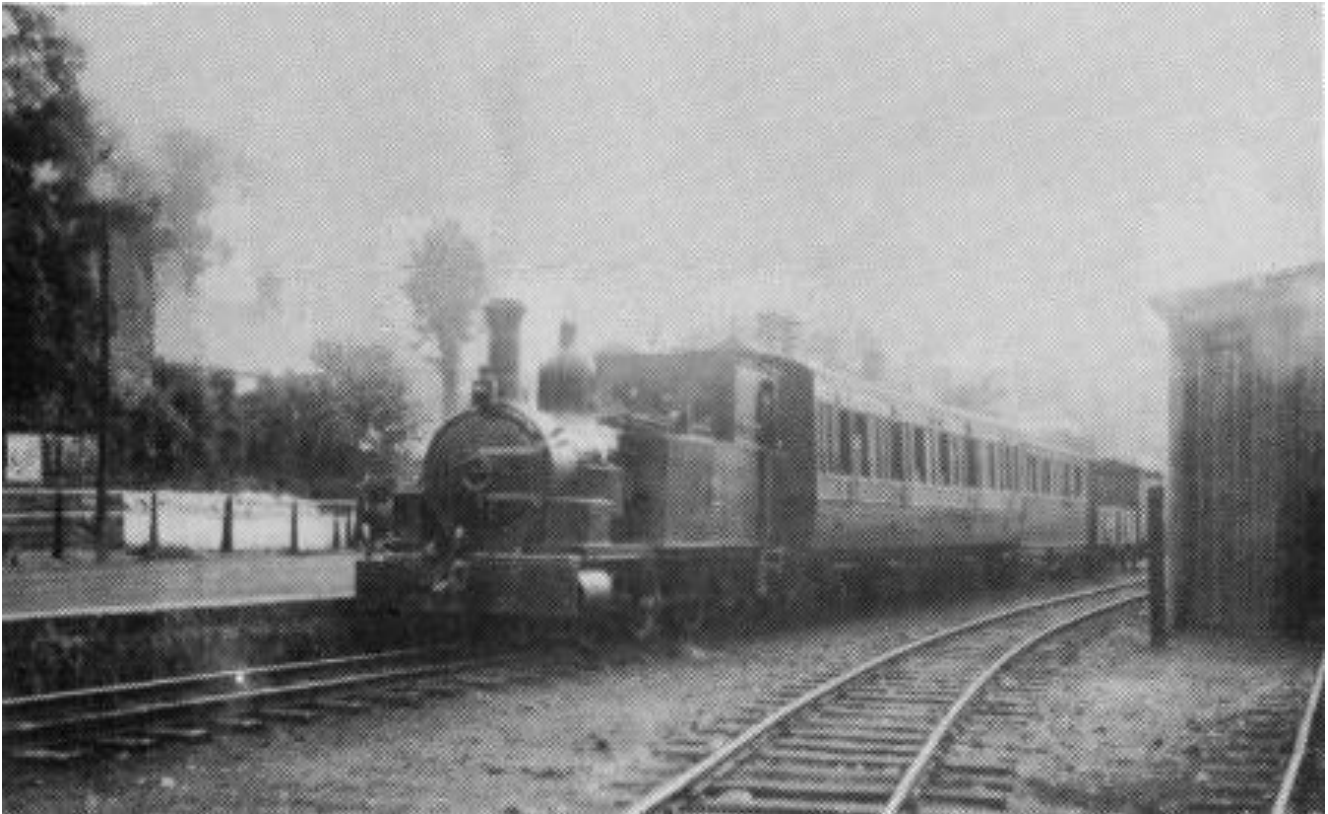
106 on train at Ballycastle. As mentioned in the article the first coach is an NCC-built centre corridor composite, while the second is an ex B&NCR 'tramcar' vehicle, built for the Cushendall road. (Real Photographs Ltd. X287
