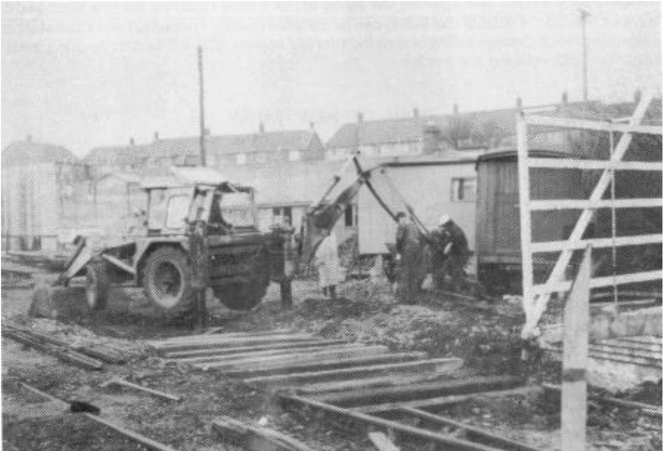
New (to us anyway) JCB digger in action laying the turnout splitting shed roads 4 and 5 shortly after arrival. (C.P. Friel)
