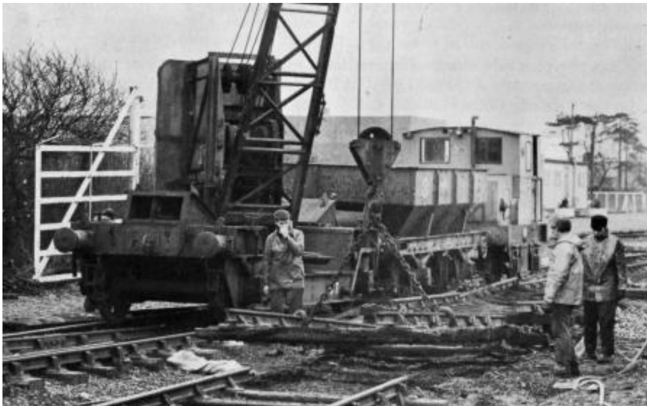
Besides moving gate posts, the handcrane which we borrowed from NIR is also invaluable for trackwork. Here it is seen lifting panels out during the relaying of No.3 shed road. Left to right are Simon Marsh, Ken Pullin and Thomas Charters. (C.P. Friel)
