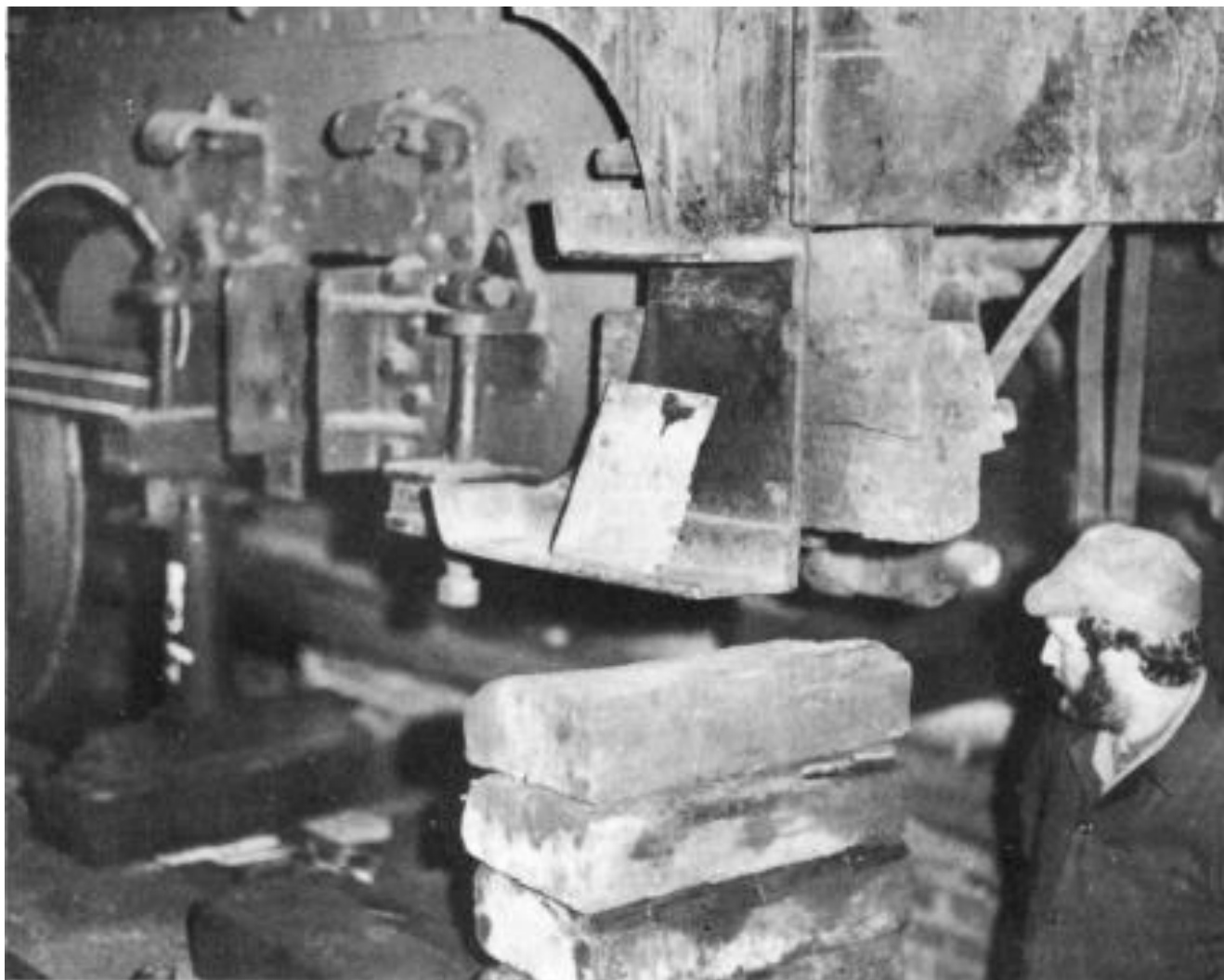
No.85's tender jacked up to allow the removal of the wheelsets for turning. (C.P. Friel)
