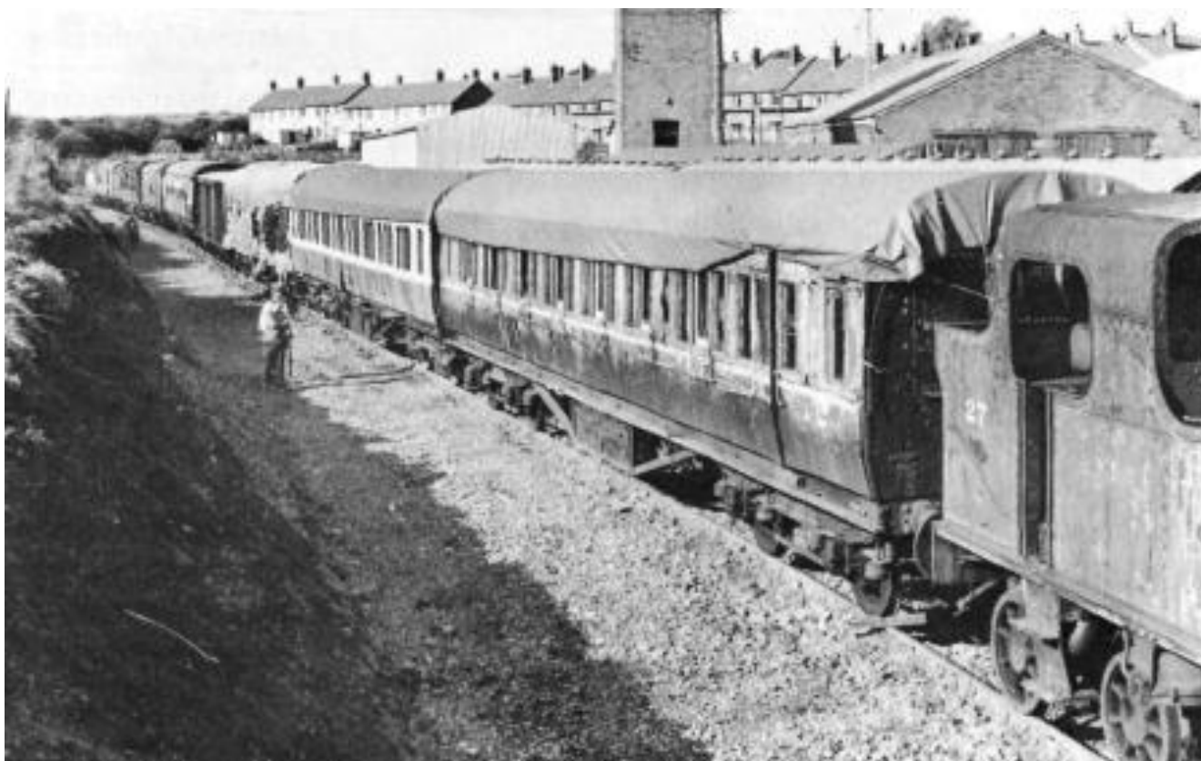
The newly excavated and ballasted trackbed for No.1 carriage siding. To the right are some of the carriages awaiting overhaul. Nearest the camera is NCC Third No.243 which retains much of its original wooden panelling. (C.P. Friel)
