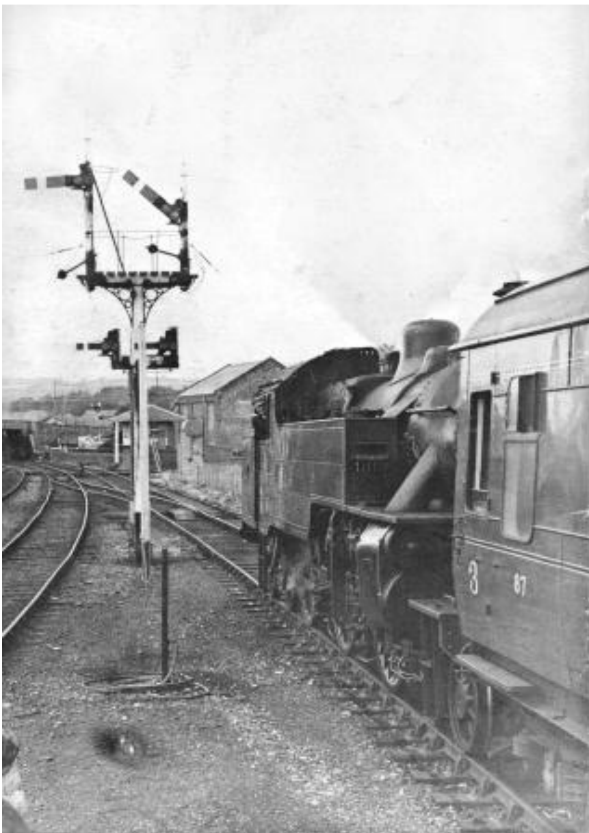
Going, going ... Inspector Frank Dunlop impatient to get away from Larne Harbour. The semaphore signals are soon to be replaced by a modernised signalling system. Larne Harbour was an isolated stronghold for LMS upper quadrant signals in Ireland, the NCC being furnished with somersault signals. (C.P. Friel)
