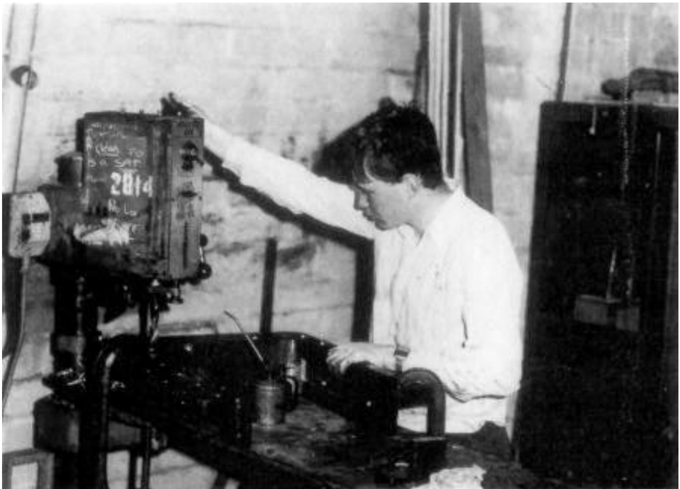
Mark Fletcher intent on getting the holes in the right places on No.461's new hornblock. (C.P. Friel)
