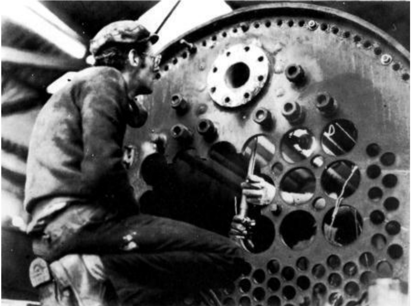
Mysterious hands within the boiler wield a cutting torch as Peter Scott studies the front tubeplate about to be removed from No.171. The photo also shows a selection of the numerous holes referred to in his report. (C.P. Friel)
