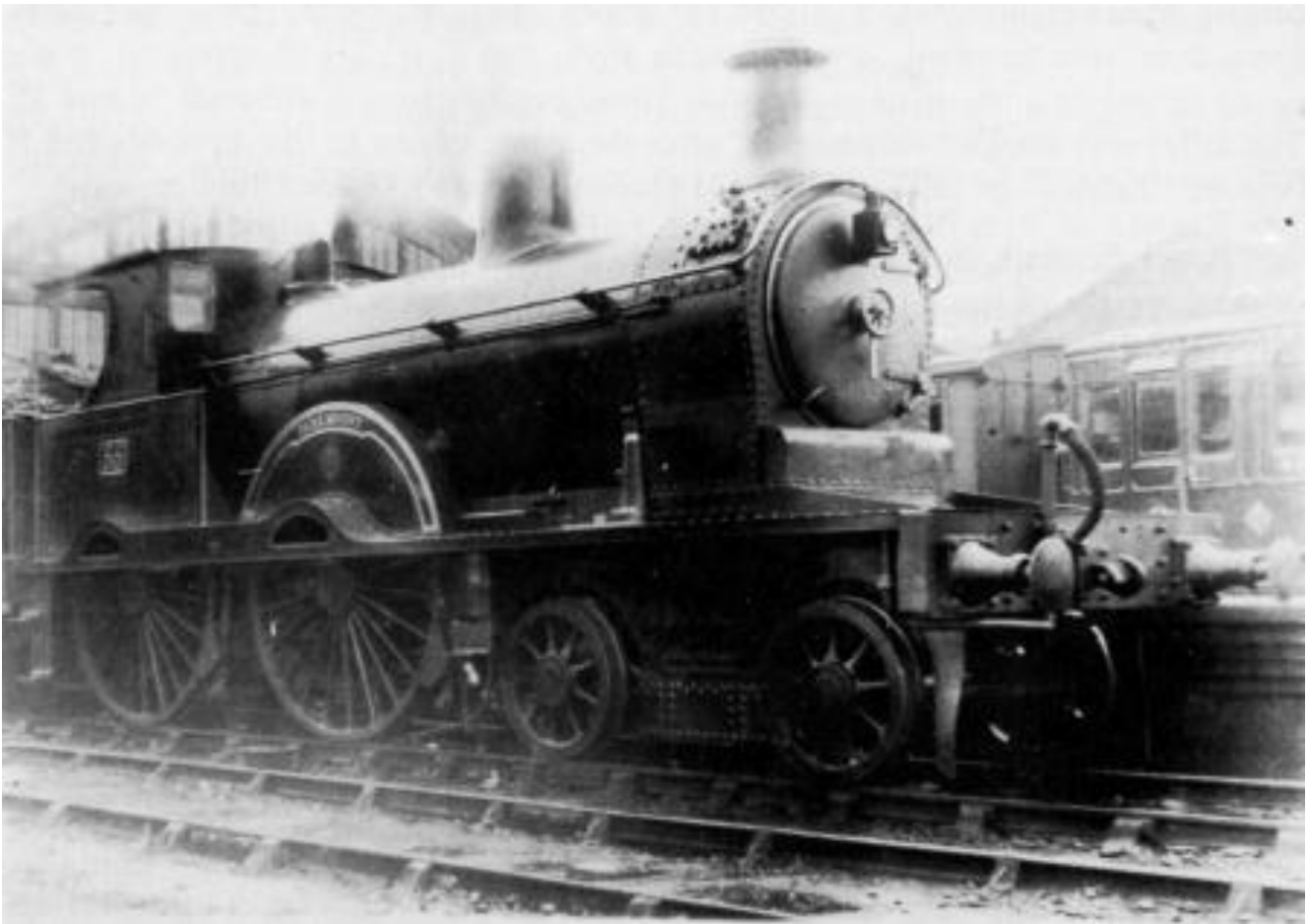
No.55 “Parkmount” at York Road in 1921, the style of chimney and splashers beading indicating her Beyer Peacock ancestry. The original station roof, destroyed in the 1941 air raids, can be seen above the locomotive’s cab. (W.T. Scott Collection)
