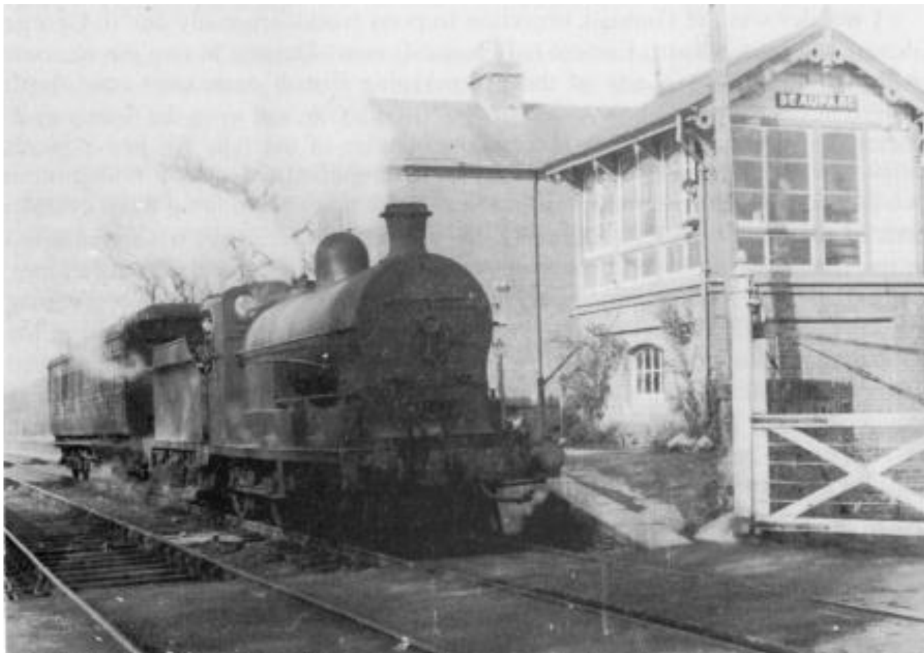
SG2 class No.17 at Beauparc with a train whose size explains the early withdrawal of passenger services from the Oldcastle branch. A fine mixed traffic engine, this class could easily run 8-bogie trains at 50-60 mph. (A. Donaldson)
