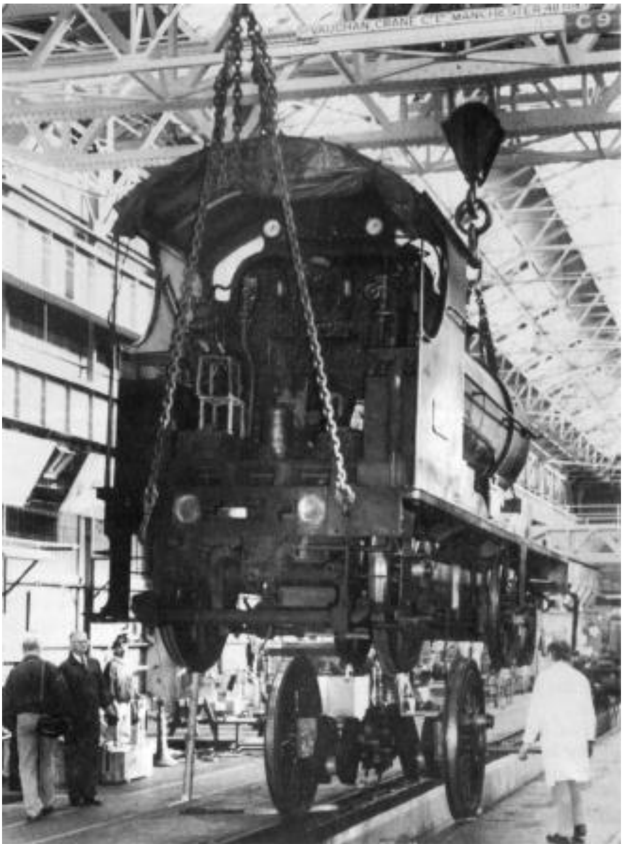
No.461 being lifted at Inchicore Works, leaving the driving axle with its offending axleboxes to be rolled away for attention. (C.P. Friel)
