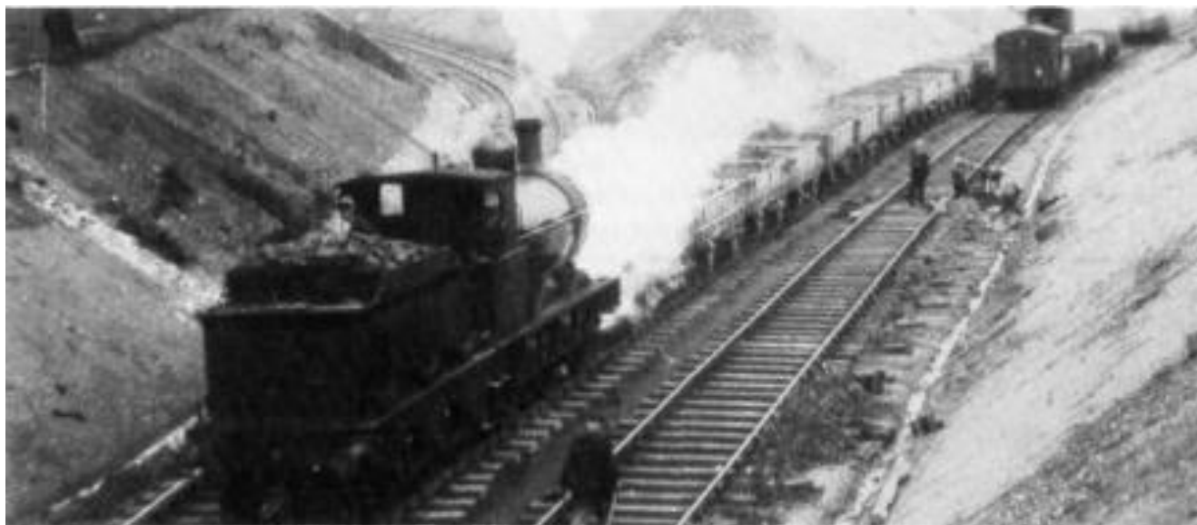
Another works train, this time at the new junction on the Belfast side of Monkstown. The new single line from Greenisland - later to be known as the Back Line - curves in from the left. The loco is No.30, a venerable Beyer Peacock 0-6-0 delivered in 1880 and rebuilt three times before being withdrawn in 1938. The date is 22 nd May 1933. (W. Robb)
