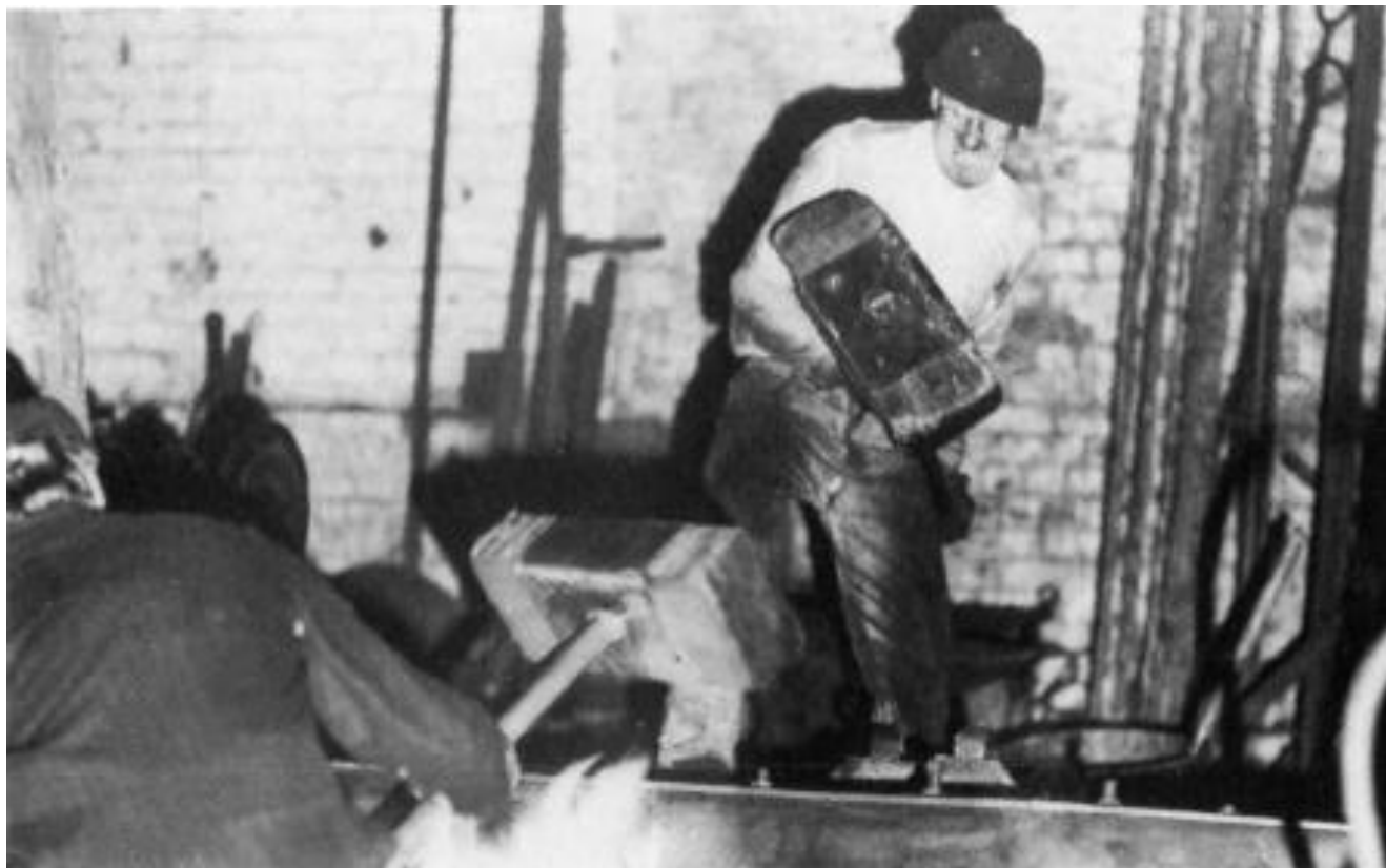
The gentle art of flanging firebox plates. Irwin Pryce on the left, in addition to the discomfort of reaching over the fire, has found that the mallet often bounces sideways after a blow has been delivered. (C.P. Friel)
