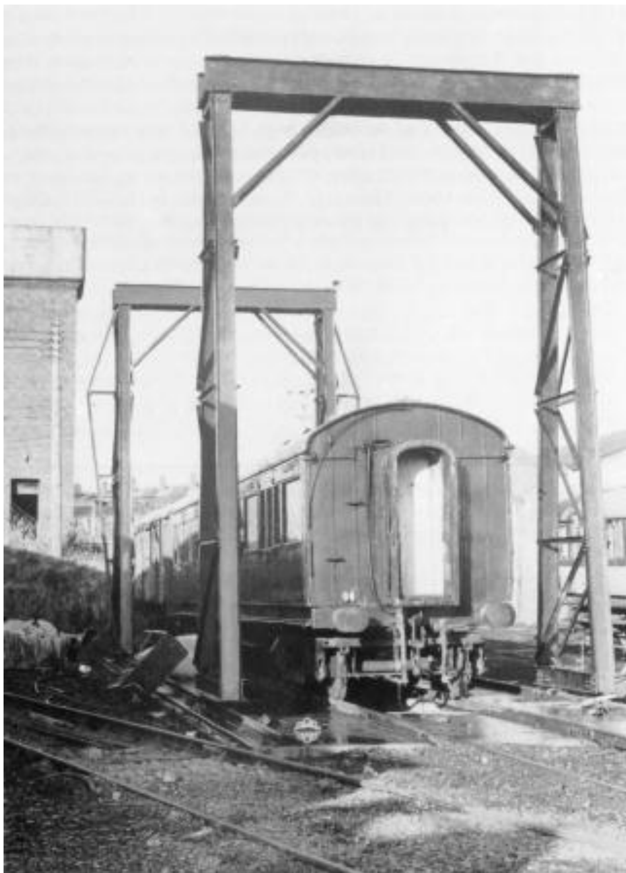
The new heavy lift area beside Whitehead carriage shed, showing the pit and the recently erected sets of sheer-legs with their lifting tackle still to be installed; 4 th December 1993. (C.P. Friel)
