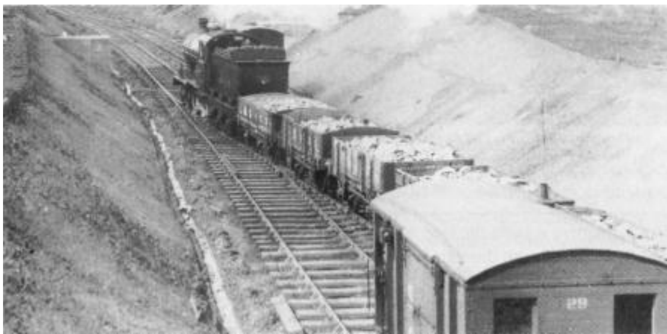
No.84 "Lisanoure Castle" with a works train on the new formation near Monkstown on 14 th April 1933. The front of the engine is near one of the siphons while the old main line can be seen in the background. Despite the direction of the exhaust it looks as though the brake van has been dropped off and a load of stone is being propelled back down the cutting. (W. Robb)
