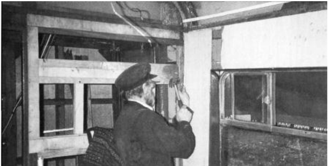
Peter Emmett replaces panelling on coach 1916 at Mullingar. (D. Humphries)
