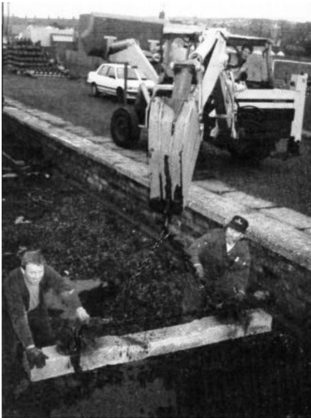
The JCB (driven by the photographer!) gets to the parts that other cranes cannot reach - relaying platform road in October 1995. (D. Mackie)
