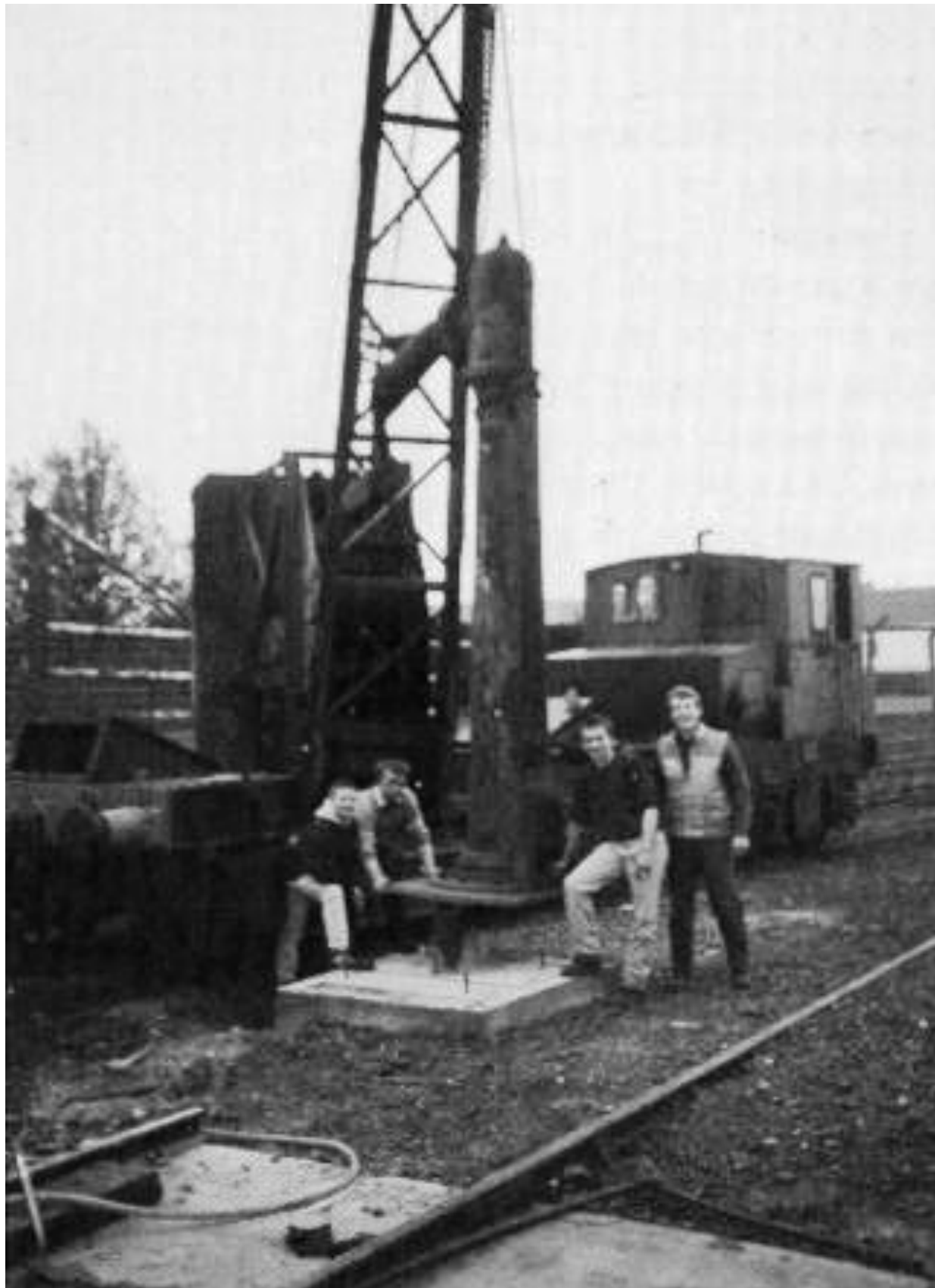
Site and C&W workers combine to install the LNWR water column at Whitehead. (D. Mackie)
