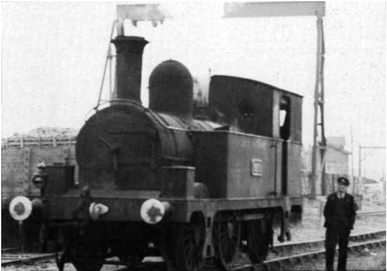
No.560 shunting the North Kerry yard at Limerick in 1957. The turned-in footsteps show that the engine has worked on the Waterford & Tramore line which had its Waterford terminus at Manor Street and was isolated from the rest of the system. Stock for the W&T would be taken to Grace Dieu Junction and then hauled over rails laid on the roadway. (W.T. Scott)
