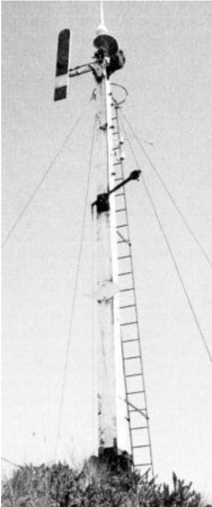
Portrush Down Outer Home signal, photographed in 1981, is approached in a cutting on a curve, hence its height. (W.P. McCormick)
