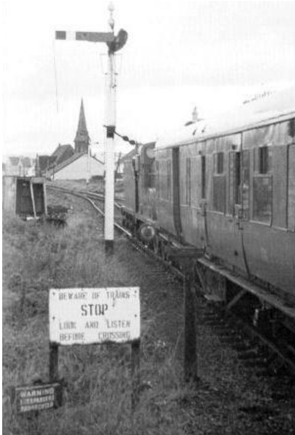
Castlerock down starter and tablet exchanger, the latter long out of use, 15 th August 1992. (N. Poots)
