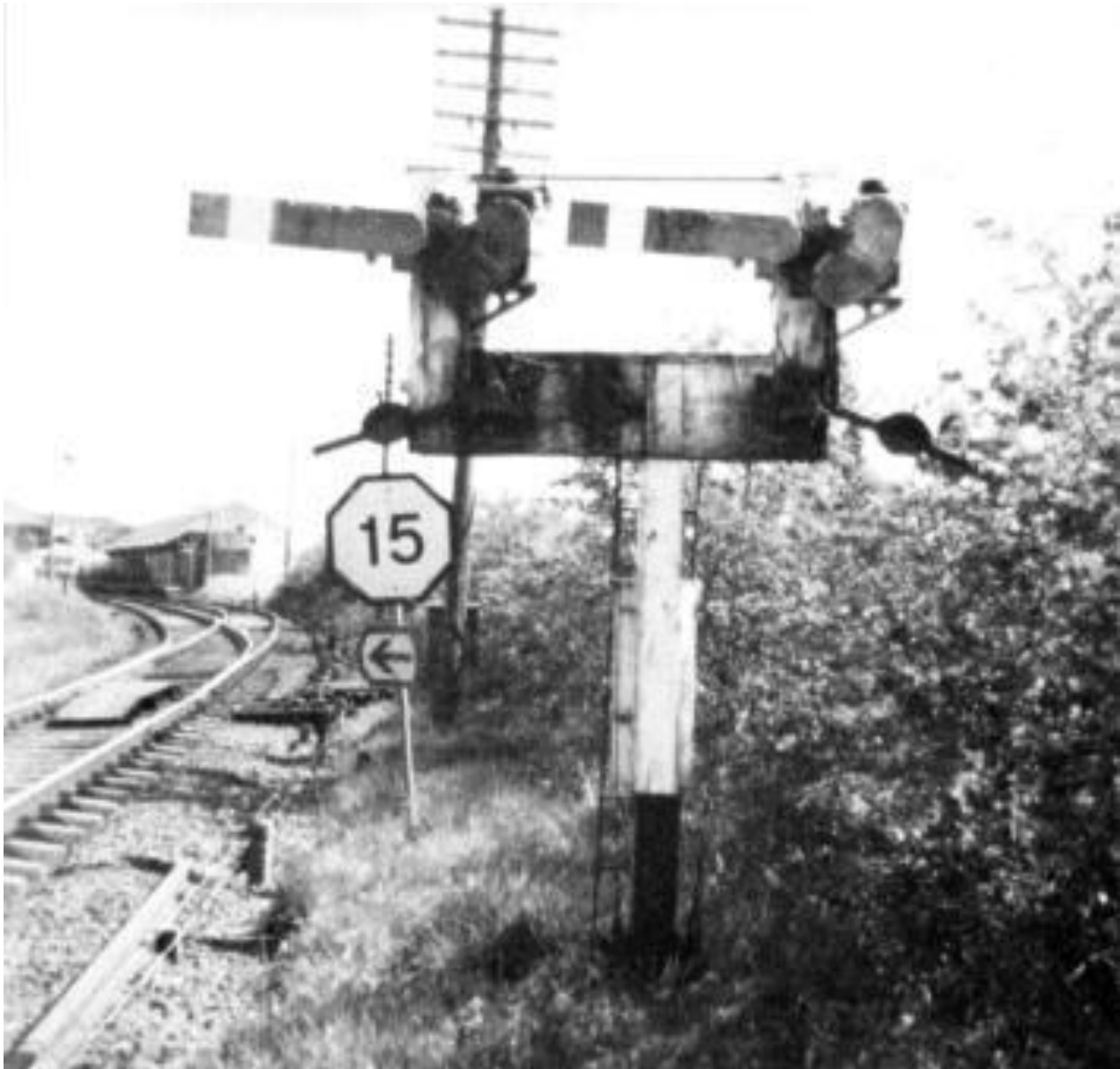
The fireman's assistance would also have been useful in sighting this stunted pair of somersault signals at the Coleraine end of Ballymoney. May 1980. (W.P. McCormick)
