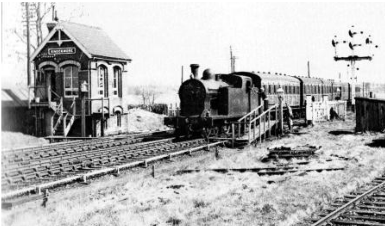
The handsome bracket signal at Knockmore Junction shows “off” for the Banbridge line as GNR T2 class No.69 collects the branch line token, 1956. (W.T. Scott)
