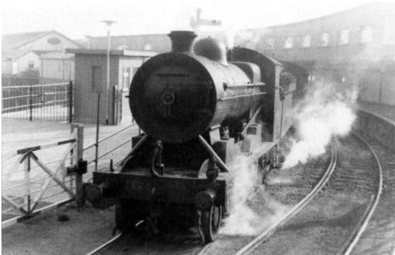
Not No.132 but No.462 with a morning boat train at Dun Laoghaire Pier station on 10 th September 1959. The pipes from the smokebox were meant to be a means of discharging ash but tended to cause air leaks. This was sometimes remedied by stuffing them with sugar beets (in season). (G. Hayes)
