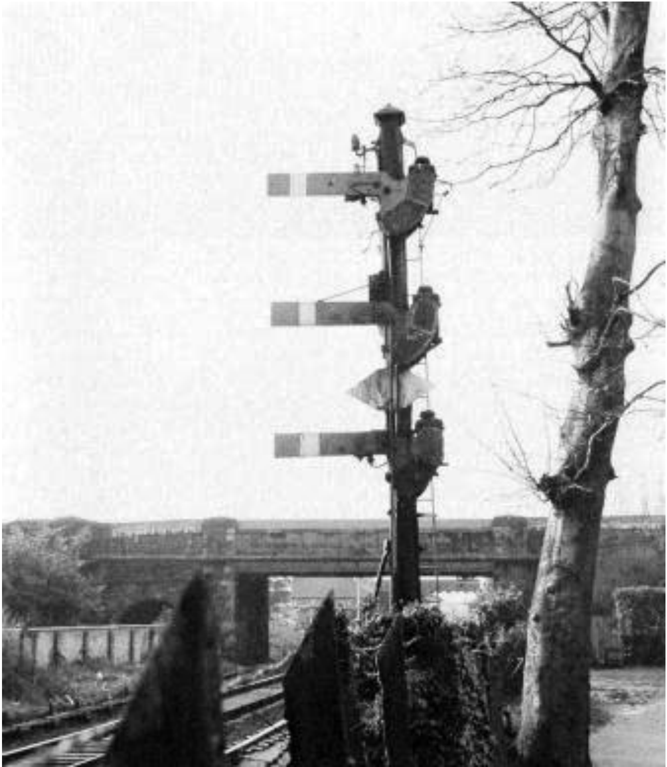
GNR 3-arm signal at Belfast end of Lisburn. (W.T. Scott)
