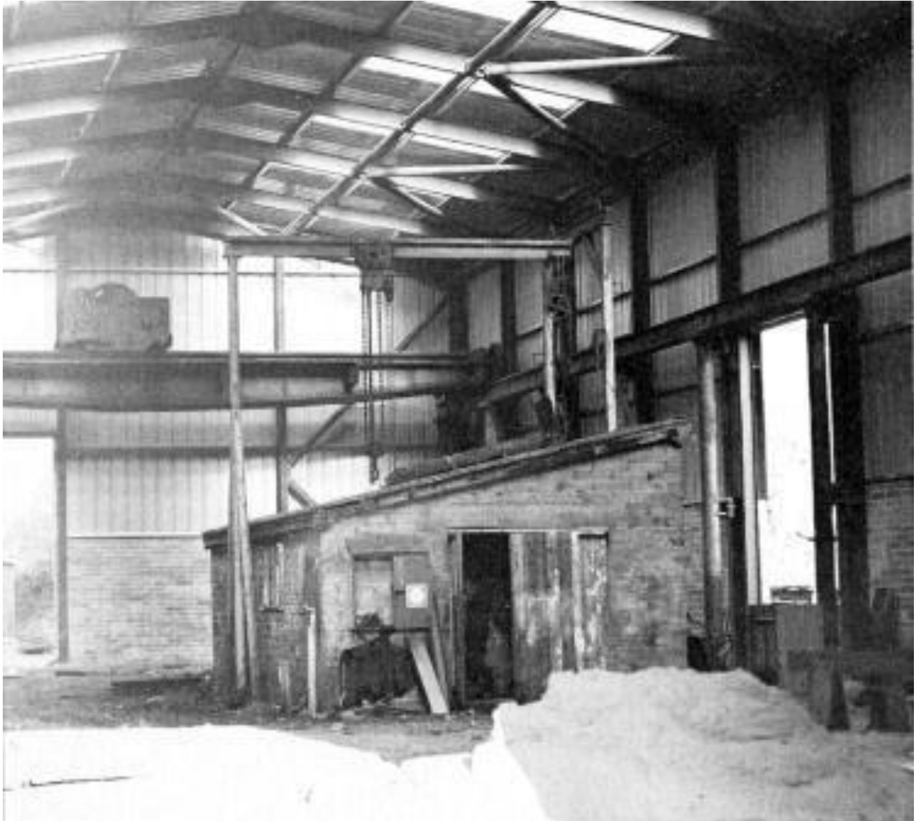
Inside the newly completed loco workshop building, looking towards Larne. The ex-Queen's Quay overhead crane can be seen in the background. The building within the building houses the wheel lathe and the gantry above it used to continue over the wheel-drop pit. (C.P. Friel)
