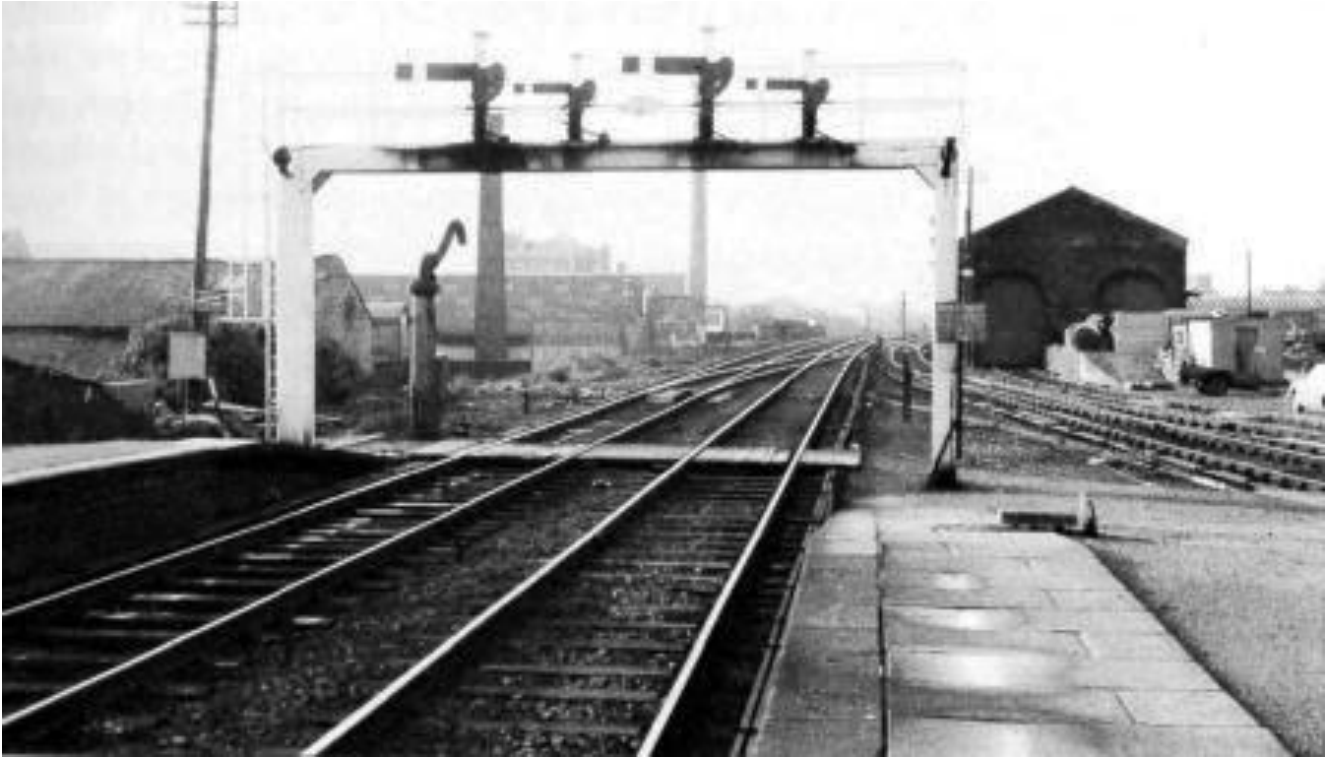
The short-lived gantry at the southern end of Lisburn. Obviously not sited with steam traction in mind, its position meant that a loco requiring water had to enter the section beyond the signal. (W.T. Scott)
