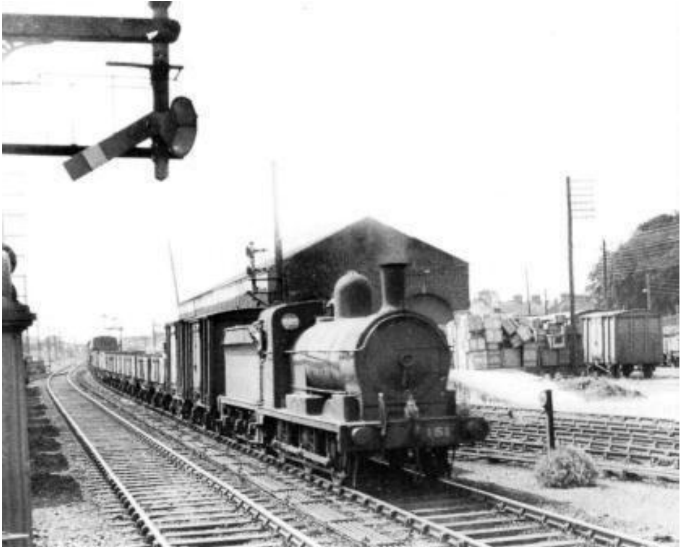
Great Northern PGs No.151 passing through Lisburn on 7 th July 1956, showing the under-hung bracket signal. (G. Hayes)
