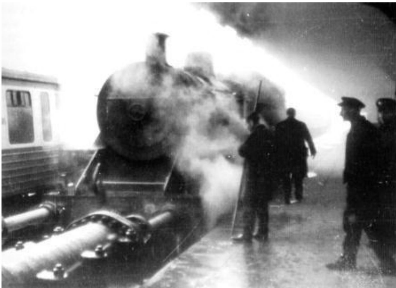
The last test of the York Road hydraulic buffers by a steam loco - No.5, on 31 st January 1970. Unfortunately a rather fuzzy photo, but the only one known to exist. (J.A. Cassells)
