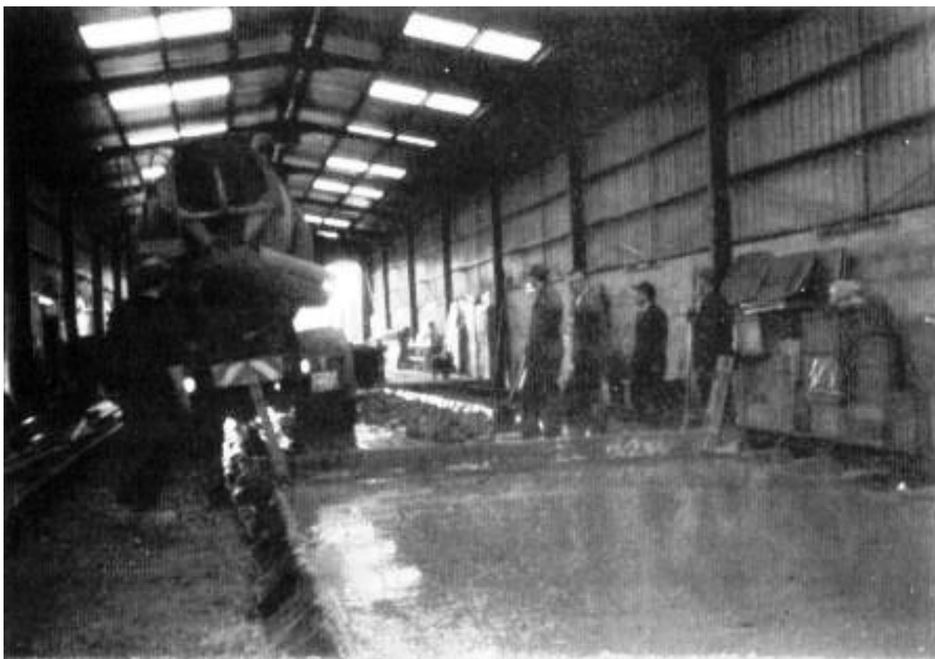
Concrete pouring in progress in the carriage shed. (J. Wolsley)
