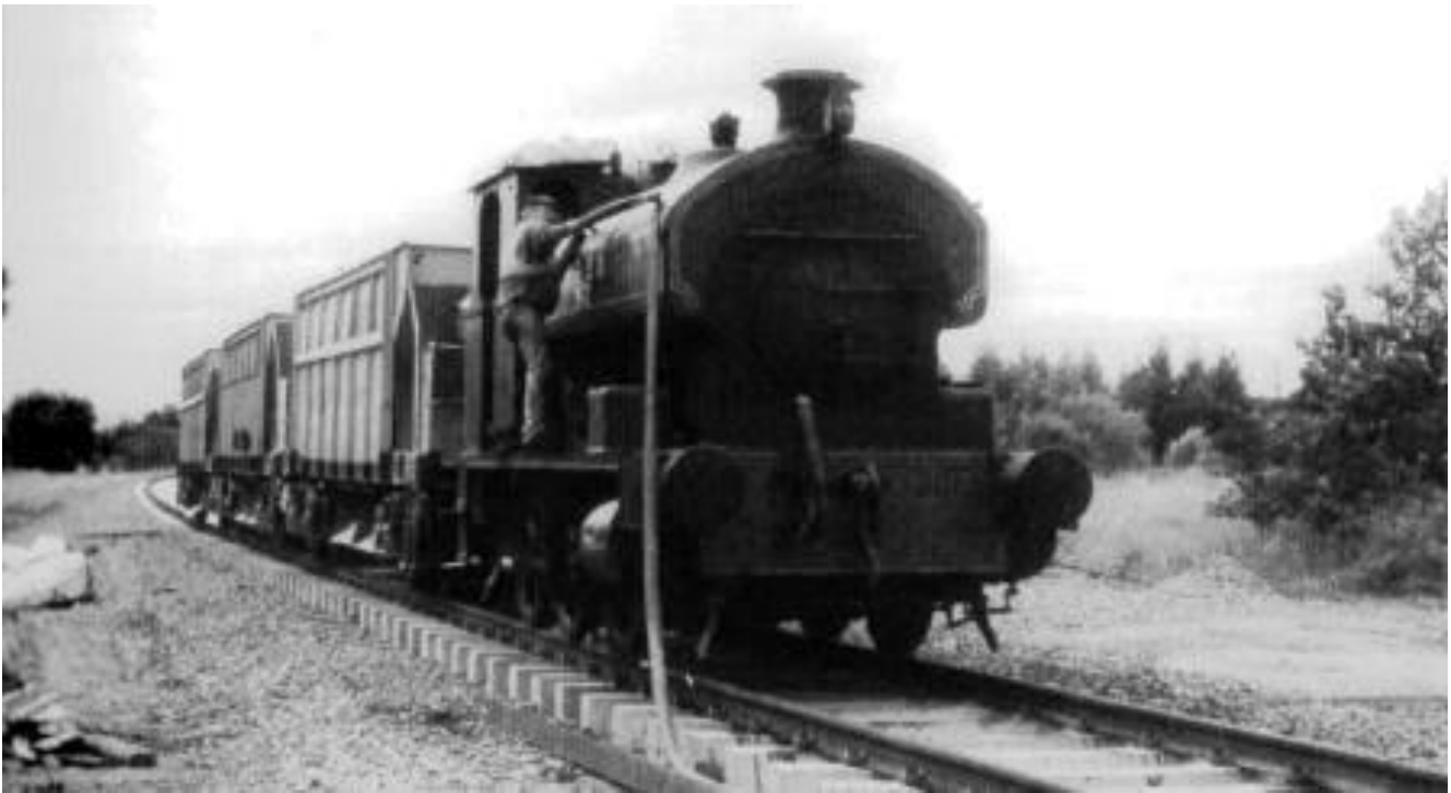
Irwin Pryce positioning the hose prior to watering at Kingsbog. Laying the hose along the handrail meant that one did not have to hang on to it to keep it in the tank and could also avoid getting soaked if the water was turned on too enthusiastically. An auxiliary supply of coal can be seen on the cab roof. (W.T. Scott)
