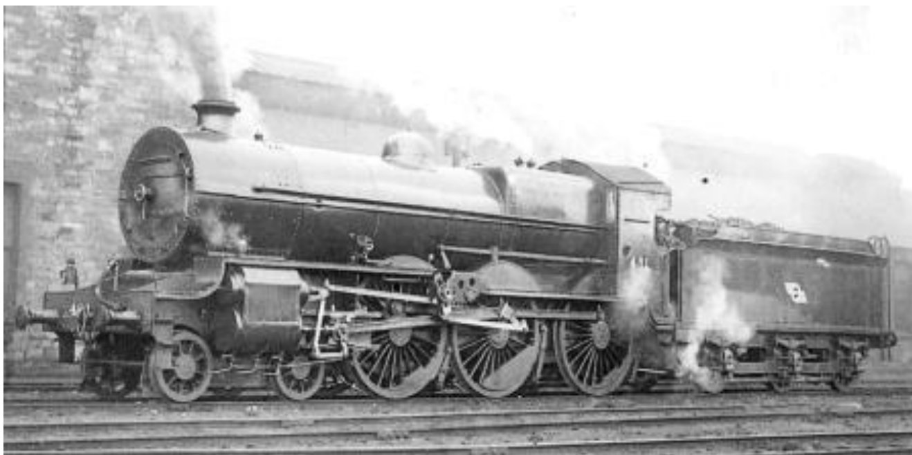
No.401, in ex-works condition in green livery, at Inchicore in 1949. Readily distinguishable from other members of the class by her different cab side-sheet with small cut-out and high handrail. (Real Photographs)
