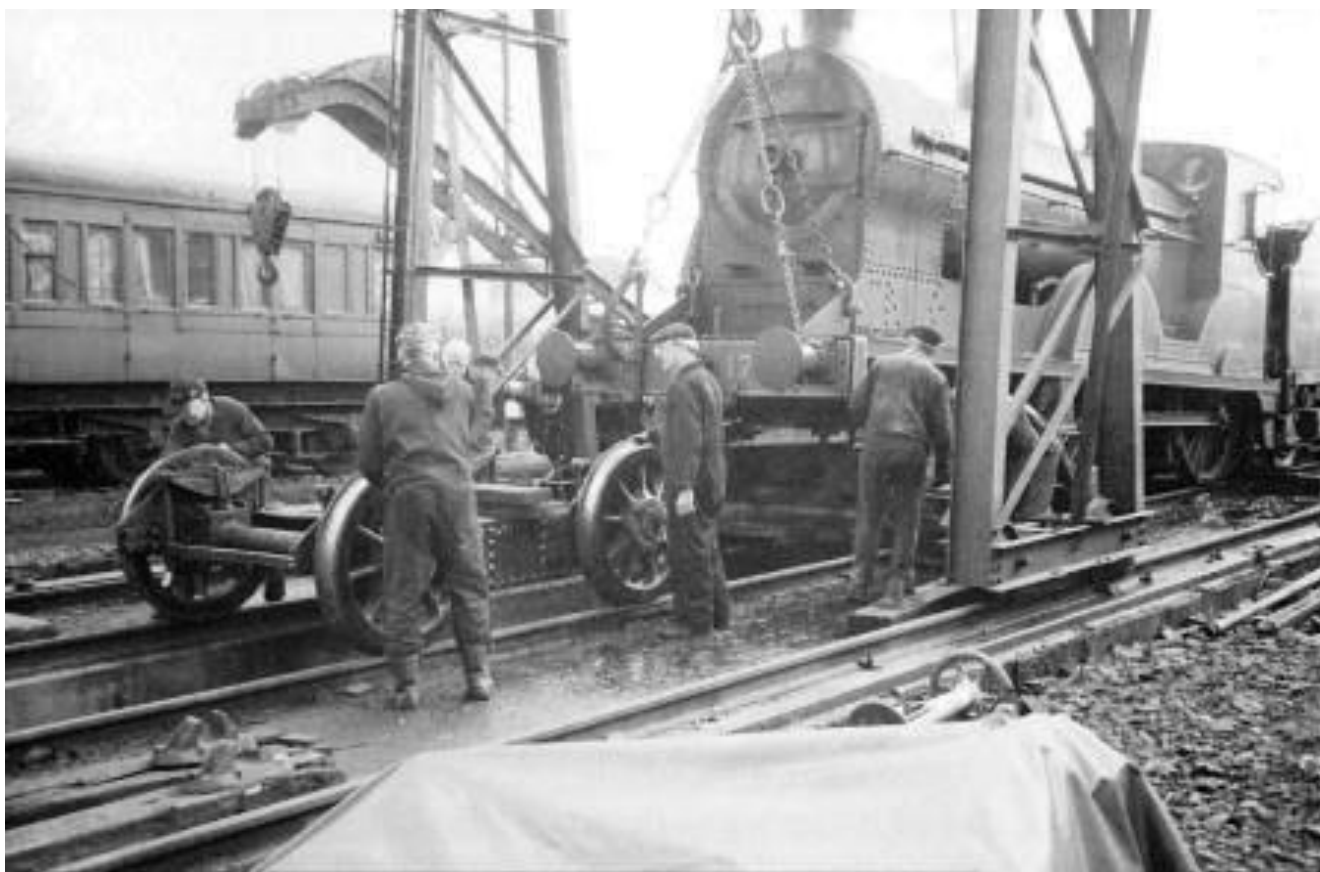
Some of its bearings having given cause for concern, No.171's bogie is removed under the sheer-legs at Whitehead. (J. Wolsley)
