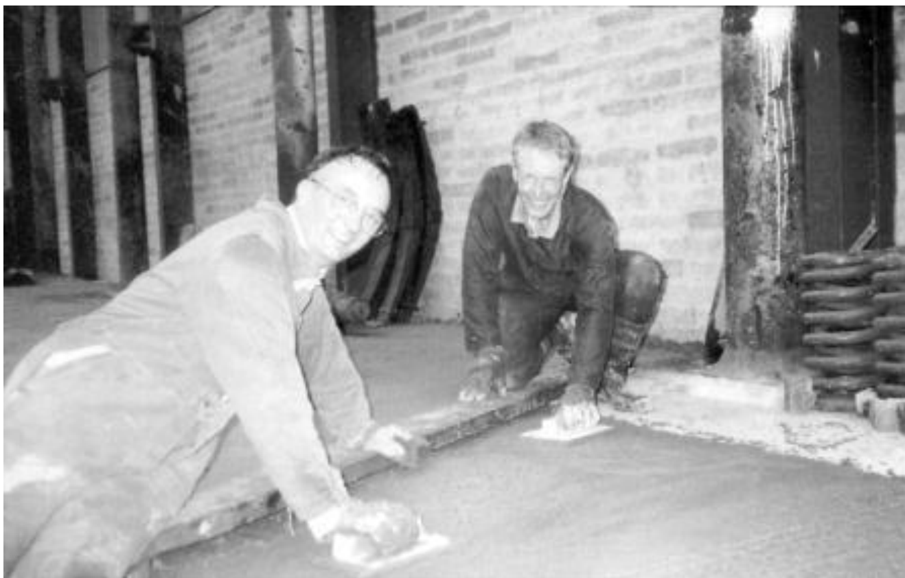
John Lockett and Dermot Mackie smoothing out some new concrete flooring in the Loco Workshop. In the corner to the left, a store with office above has since been constructed. (J. Wolsley)
