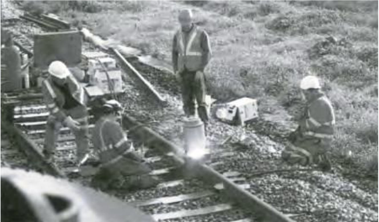
The Thermit welding team in action. Since they are at Greenisland it will be some weeks before shellfish become available. (I. Pryce)
