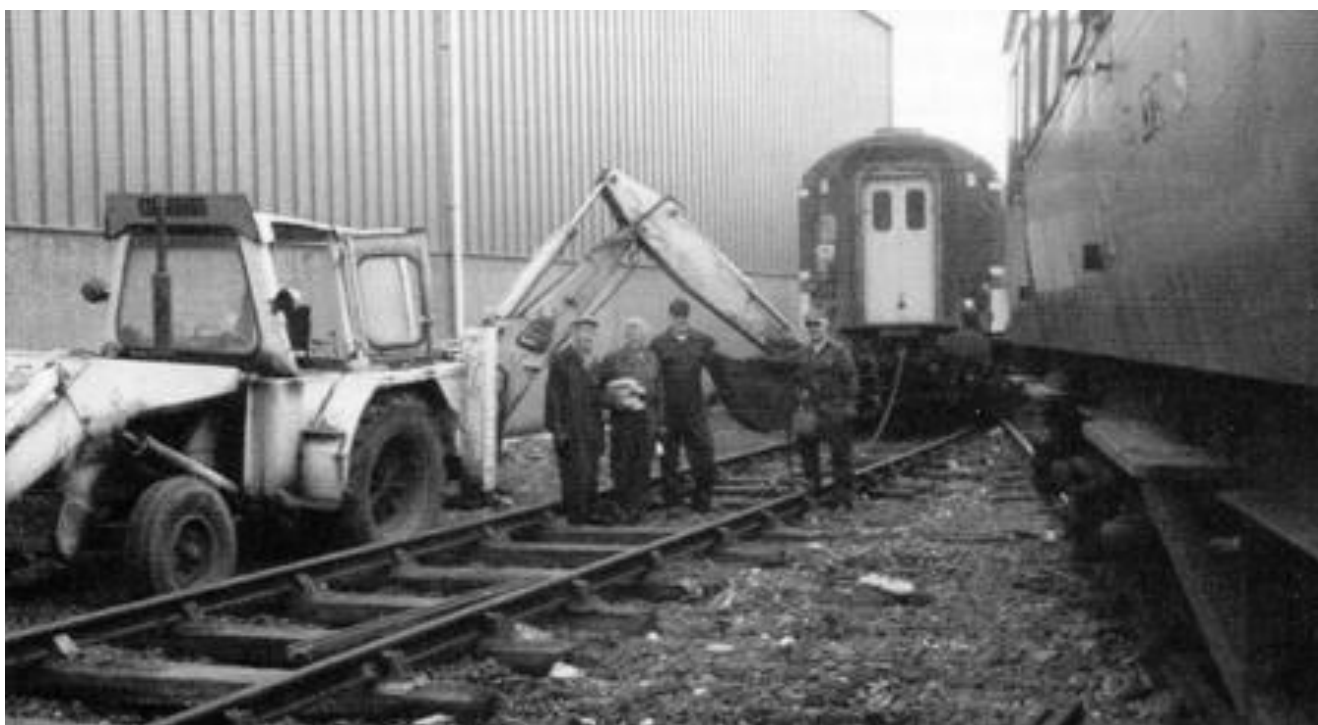
Dermot Mackie and Site Gang members Alan McRobert, Paul Wilkinson & John Williams. The multi-function JCB is about to pull the Mk3 sleeper coach out of the newly connected fifth carriage road. (D. Jenkinson)
