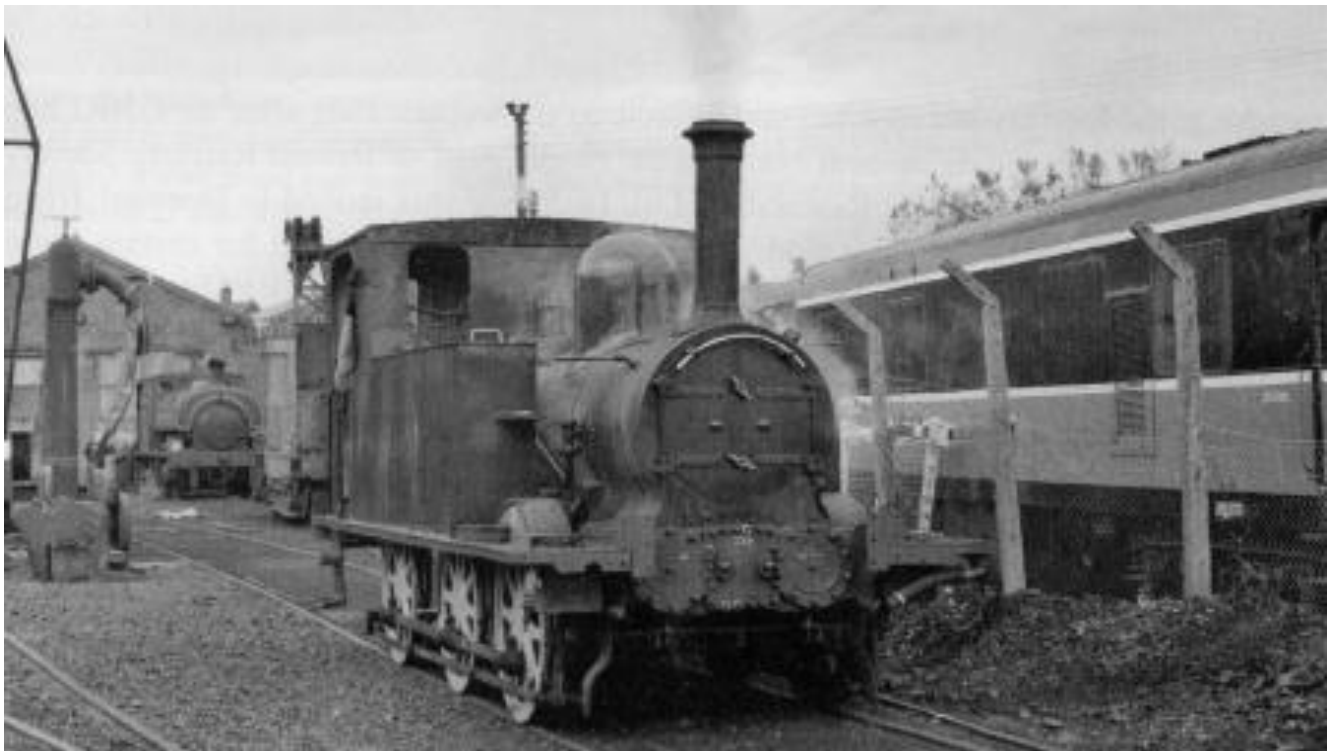
With the Guinness engine in the background, the diminutive No.90 ventures forth after attention to her valve gear. The front buffer beam has been removed to provide access. (I.C. Pryce)
