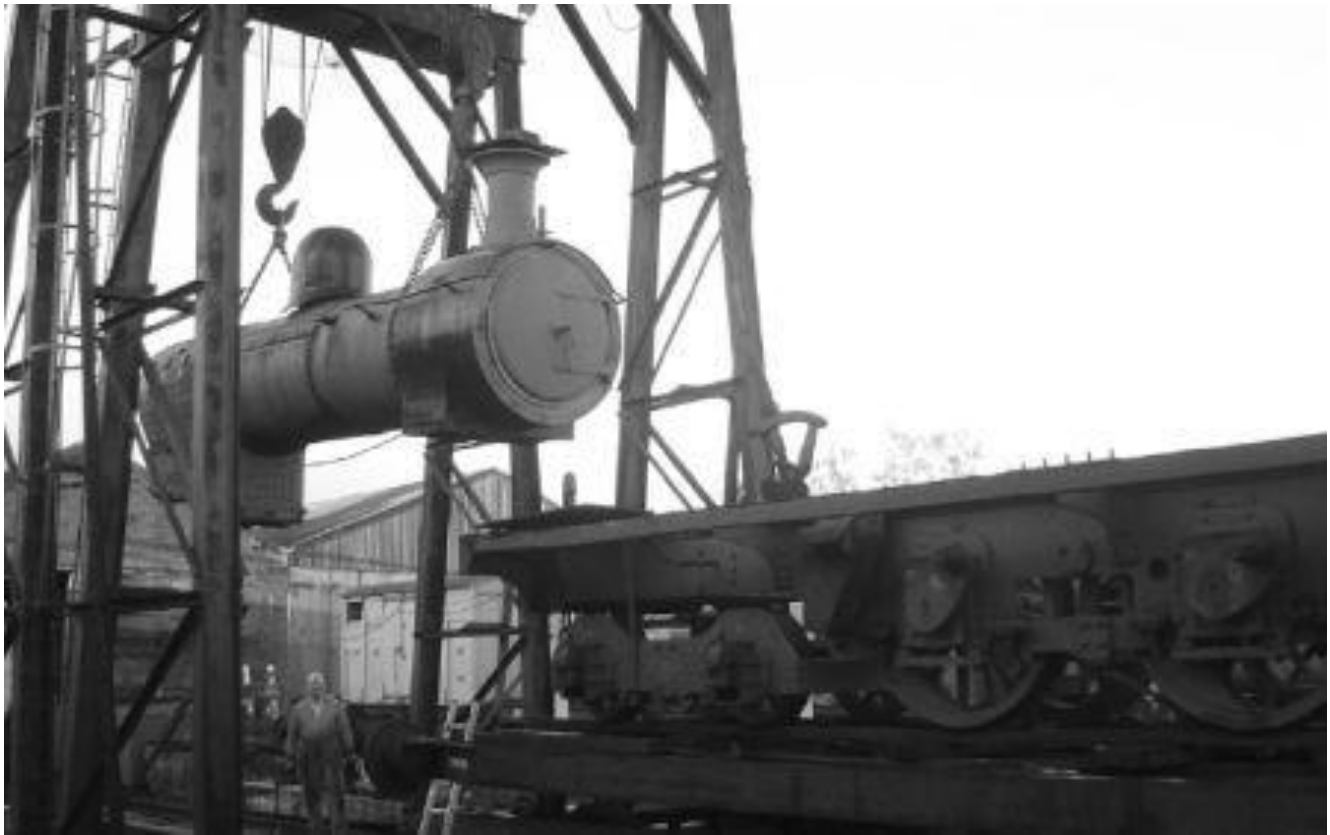
The boiler of “Drumboe” is lifted out of the frames prior to being placed on works trolleys. (J.J. Friel)
