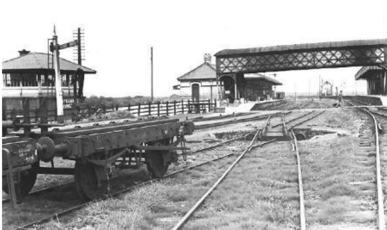
GNR tranship wagon 26 at the mixed gauge turntable at Strabane. (C.H. Hewison / S.A. Leleux)
