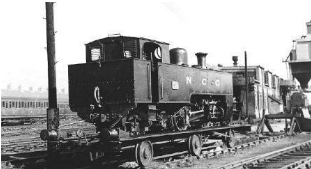
NCC 2-4-2T locomotive No.42 on the 6-wheel transporter wagon 3094 at Belfast York Road on 17 th April 1948 - probably the loco's final Works repair. (H.C. Casserley / S.A. Leleux)
