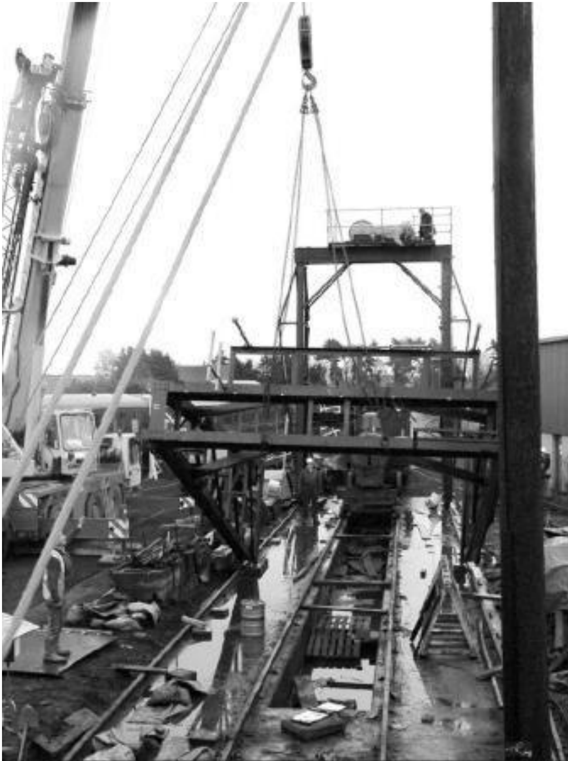
Re-erection of the sheer-legs on a rather wet 22 nd November 2008. The set at the Belfast end, and its winding gear, have been restored to their rightful position and the road crane is now lifting the other set. The pole which had a narrow escape is on the right. (A.C. Ragg)
