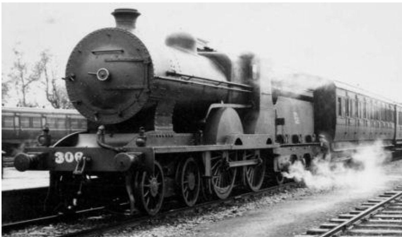
D12 No.306 at Limerick Junction, date unknown. Although there is provision for eight "dogs" to secure the smokebox door only five are in use - probably still preferable to wrestling with the original dart and shiny ring. (A. Donaldson/W.T. Scott)
