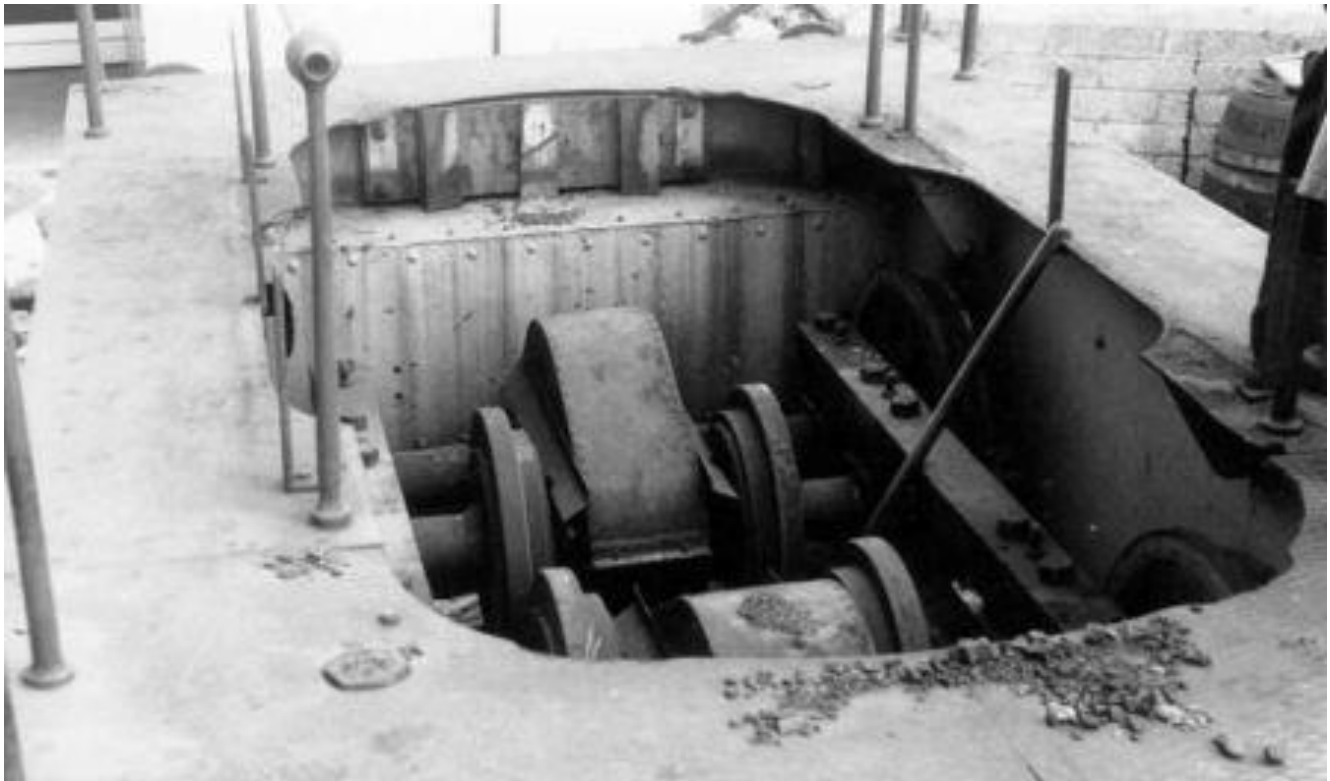
A Guinness transporter wagon photographed in June 1964. The housing containing the gearing to the wagon's wheels can be seen, as can the rollers on which the narrow gauge loco's wheels rested. (H.C. Casserley / S.A. Leleux)
