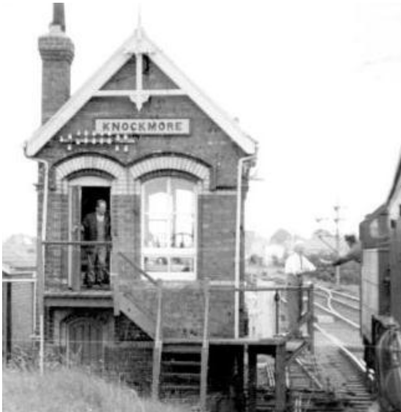
On 12 th July 1965 fireman Foy, on the 11:00 special from Antrim, gives up the token for the Antrim-Lisburn section. Following the first closure of the branch to passenger traffic in September 1960 a Tyer's instrument replaced the former staff section to Ballinderry. (J.A. Cassells)
