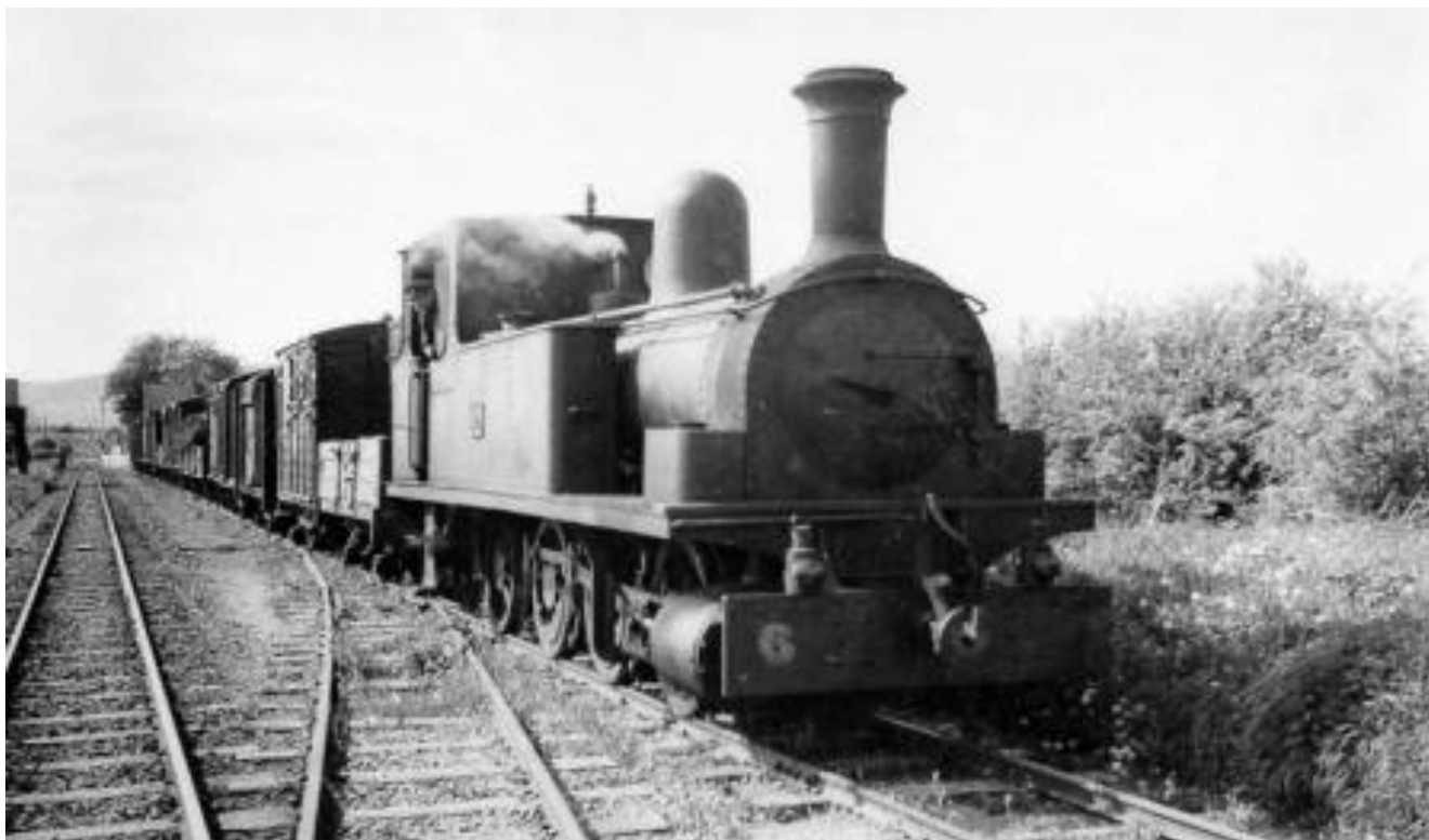
West Clare 0-6-2T No.6 with a goods at Corofin in 1950. The trailing wheels on these engines were originally the same diameter as the drivers but this was found to be hard on the track. Increasing their side play failed to cure this and the trailing wheels were eventually reduced in diameter. (Kelland collection / W.T. Scott)
