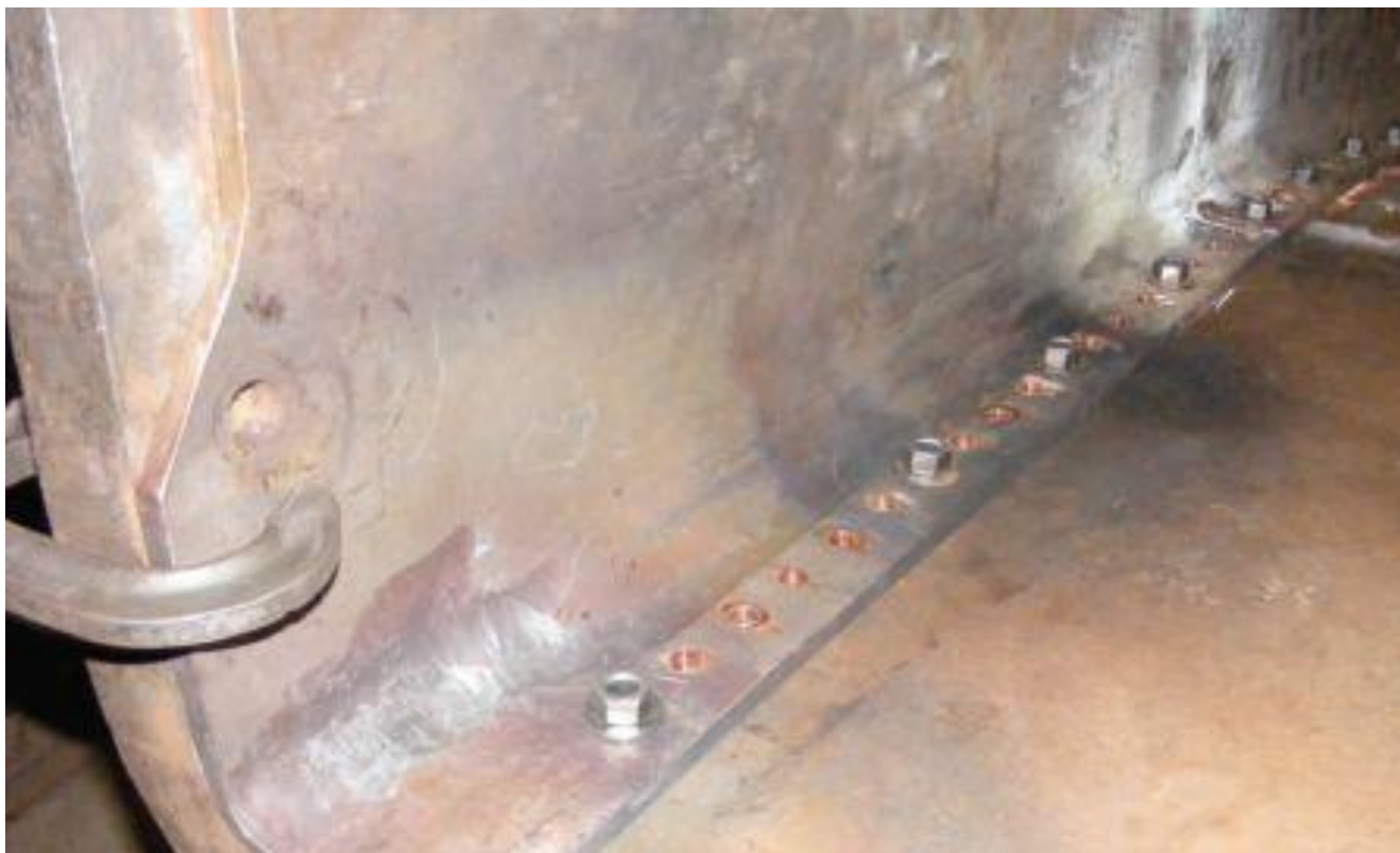
Trial fitting of the new inner firebox plates for No.461, 10 th August 2009. (C.P. Friel)
