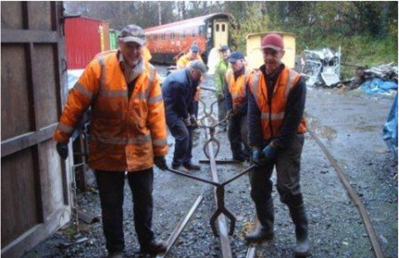
Laying the extra rail for 3ft gauge into the workshop, 17 th November 2010. (D. Mackie)
