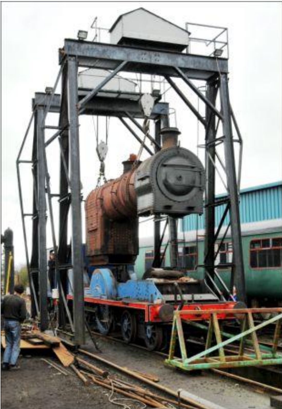
No.171's boiler emerges from the frames on 23 rd February 2012. (J.J. Friel)
