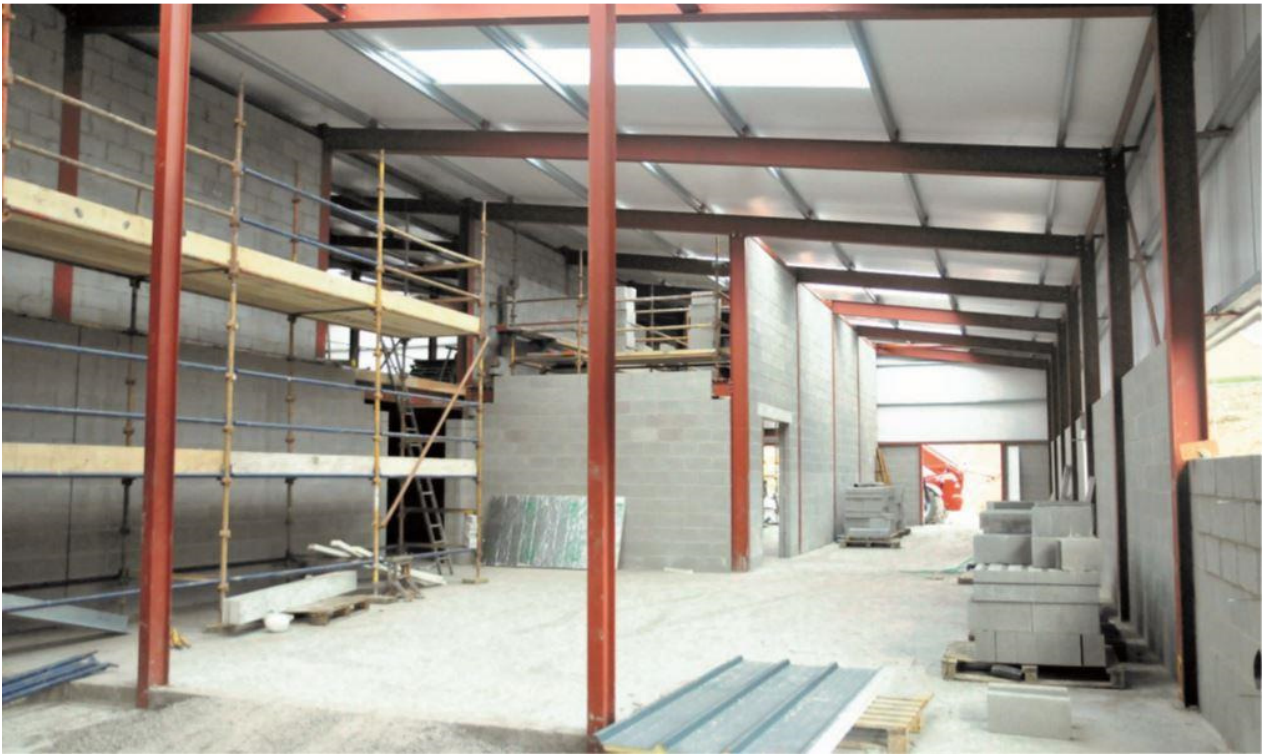
Inside the new workshop building currently under construction beside the wheel drop shed. Behind the wall to the left is a new machine shop; on the floor above, the new changing and canteen facilities, replacing the venerable 'Tarry'. In the centre of the picture, the walls around the new foundry are going up.
