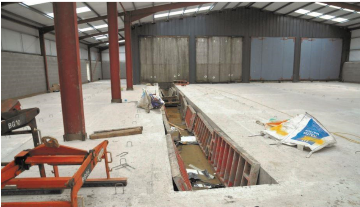
This was the view in January 2016 facing Belfast, with an inspection pit in place under road 'D'. As we go to press, the temporary wall with the 4 doors has now been removed and a new partition is being built to divide roads C and D. The area to the left is the carriage machine shop, which will contain tools for the overhaul of carriages in road D. A viewing area at the far end to the left will allow visitors to see the workshop in action.
