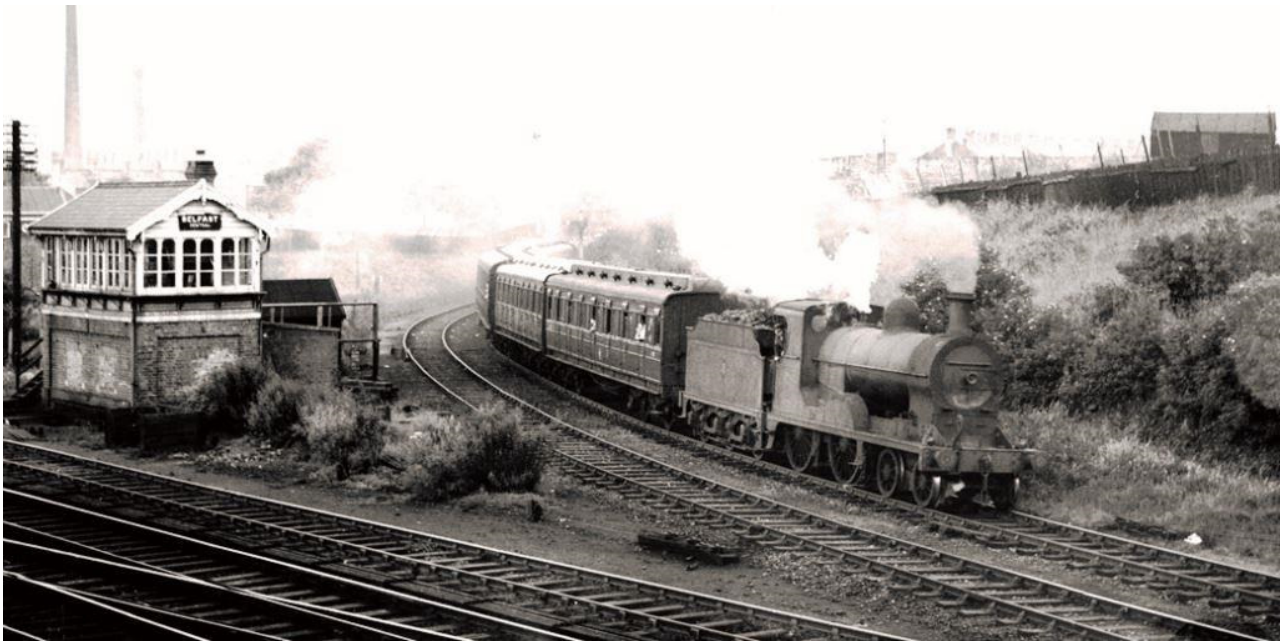
Early in the summer of 1959, UTA No.64 Lough Gill (GNR(I) No.196) passes through Belfast Central Junction with a Bangor to Dublin Excursion. As on the 1938 occasion mentioned in the text, the engine is paired with a higher capacity tender than was usual for the U class, a 3,500 gallon type D1 or D2. (A. Donaldson)
