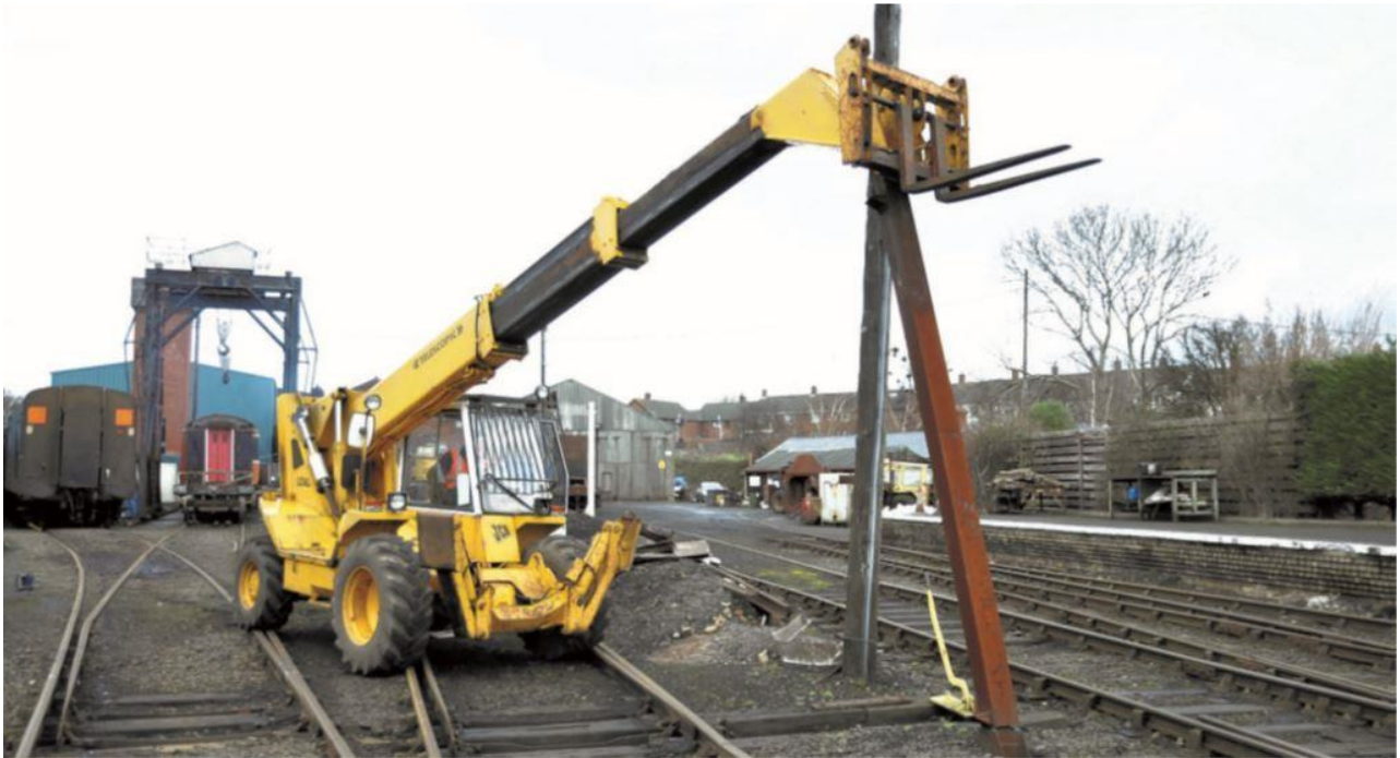
The Telehandler assists with the removal of a redundant gatepost on 20 th January 2015.
