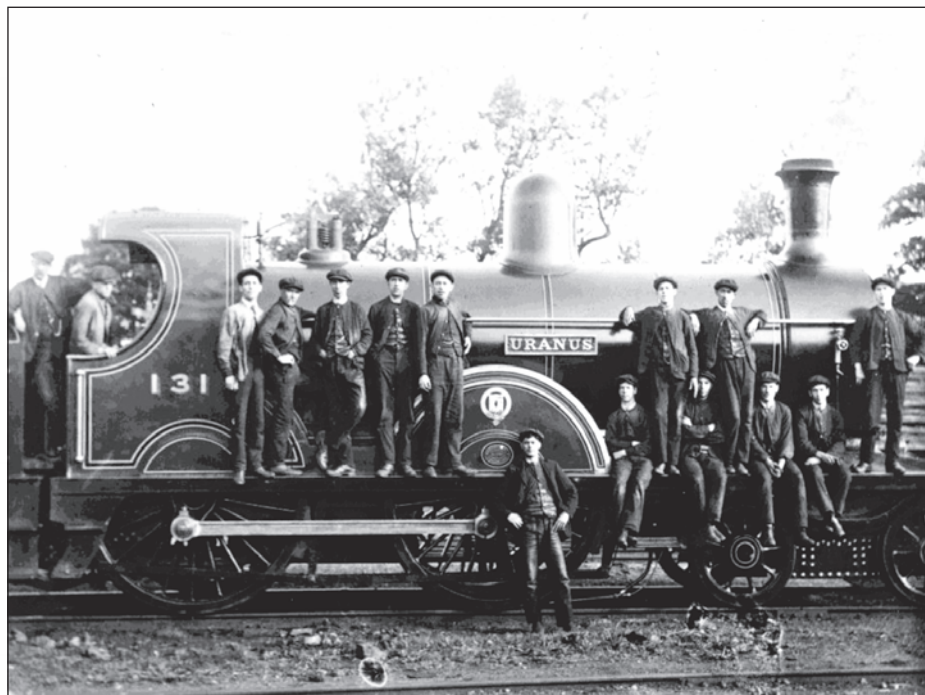
No.131 in original condition with green livery and low boiler - and hence longer chimney, seemingly not made from one casting - has attracted quite the crowd of fitters and / or shed staff for this very early C20th photo, perhaps at Dundalk shed. The "Uranus" (Greek god of the sky) nameplate is prominent but nameplates, like blue livery, were not applied to the re-built form of Q we now have, which is one reason No.131 does not now carry them. (Photo: C Friel collection)
