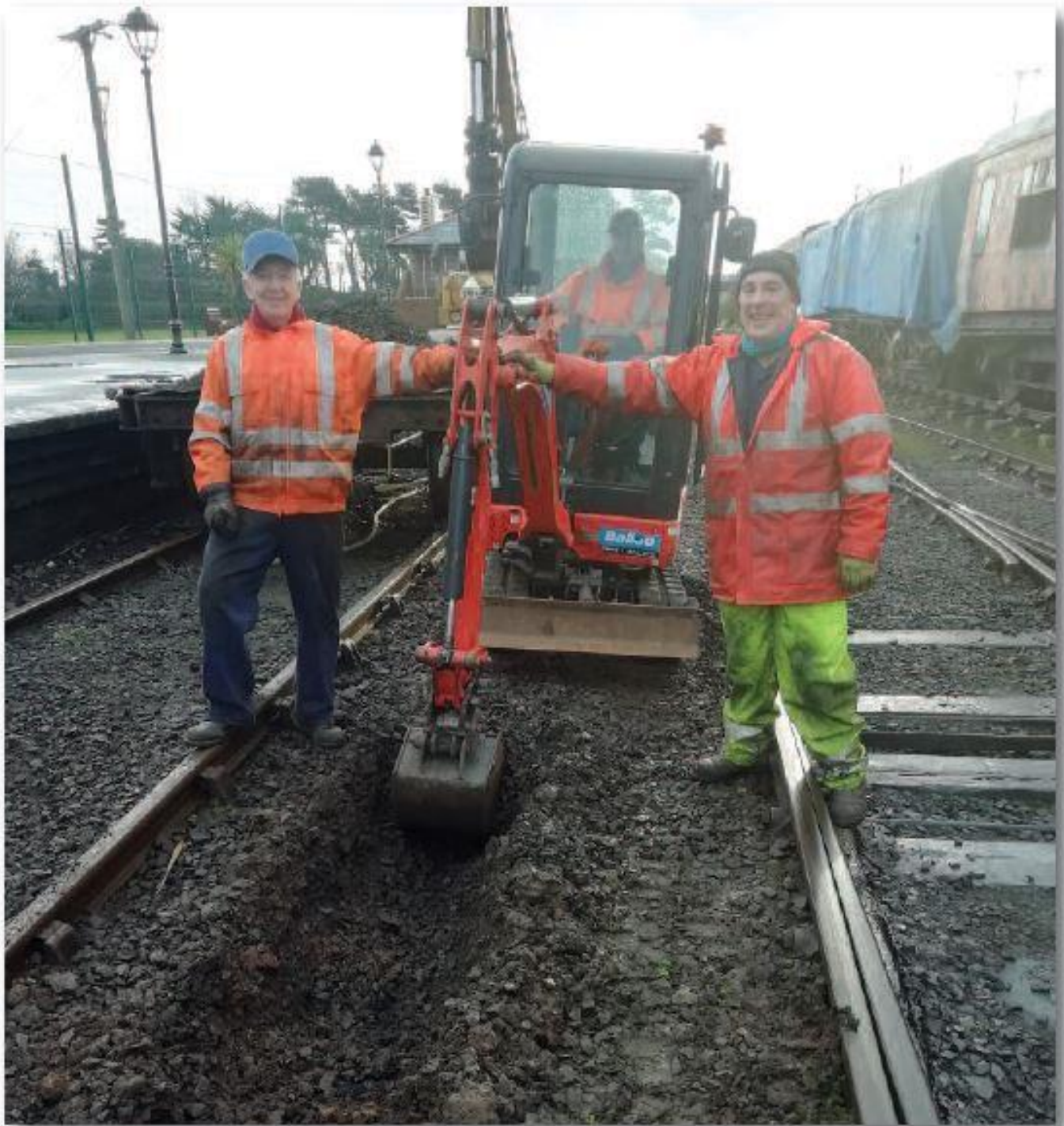
Tom Mathers and Colin Stewart flank Dermot Mackie, in a hired in digger, as they start to dig a new drain between the platform and loop roads on 07th January. The results were both instant and exceptionally good. (Photo: G Hunt)
