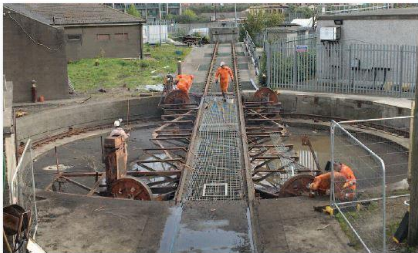
During: Spring 2020 and the filthy, somewhat oily, pit has been cleaned out, the obstructive fence on the right has been moved back from the brink and work progresses on the table itself.
