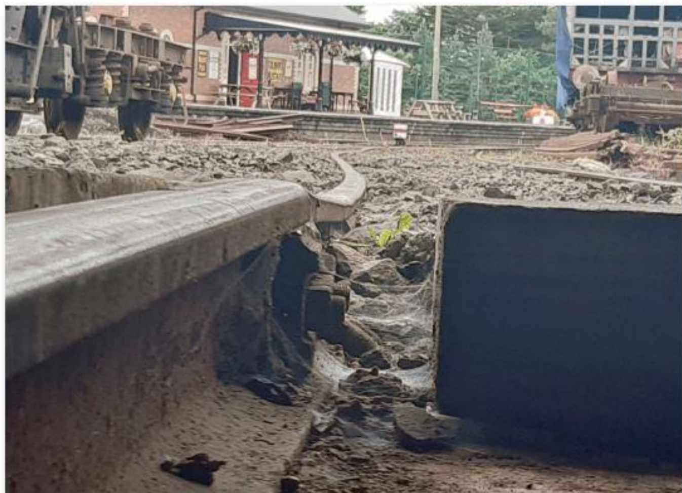
One of the major bugbears both of the Carriage Officer, whose buckeye couplings and nerves it strained, and steam loco crews whose gauge glasses it unexpectedly drained just as they buffed up to carriages, was this change of gradient at the shed door in A-Road. After a few more restrained attempts failed to correct it, in October the Site Squad essentially tore it up and raised the lot, all the way out to the junction with B-Road. (Photo: J Friel)
