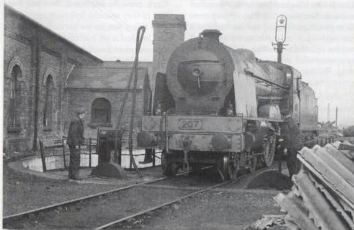
VS Class No.207 'Boyne' on Amiens Street (now Connolly) turntable in the 1960s, still facing into the terminus. The table had the option to vacuum operate, via use of the loco's brake ejector.
