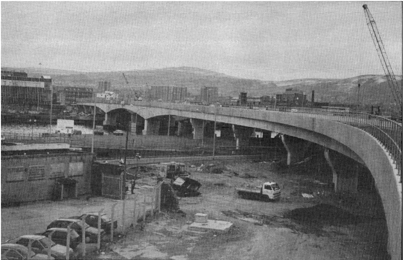
Dargan Bridge, Cross-Harbour Rail Link Belfast, April 1994.
