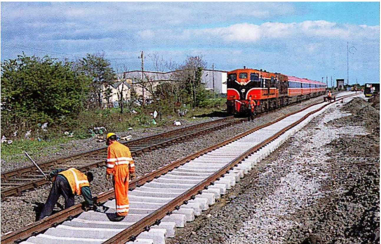
Renewal of the Down road in progress at Liffey Junction, 20 th April 1997. (15:45 Connolly/Longford passes on the wrong road.)
